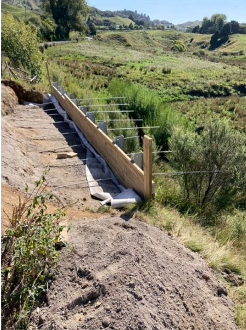
Figure 3: RP2.97 - New steel columns installed replacing the old railway irons
