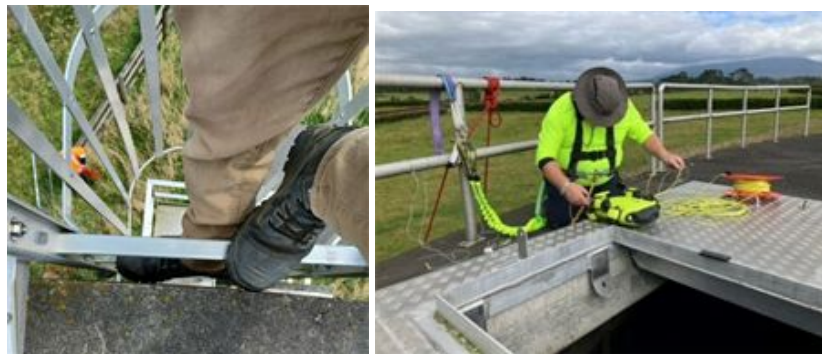
Figure 5: Inspection in Progress
