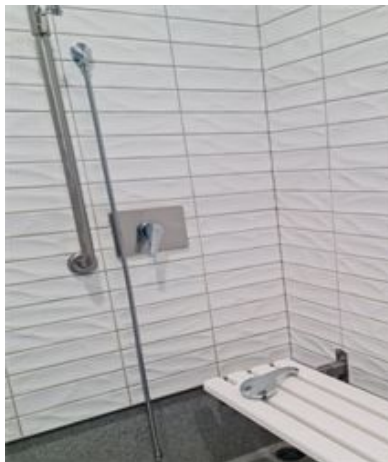
Figure 16: Photo pf Wai o Rua shower replacements
