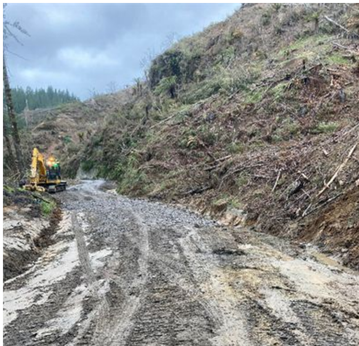
Figure 45 - Photo of Mangaoapa Road
