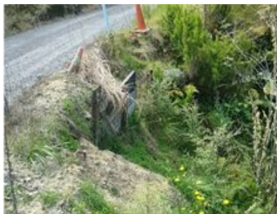
Wall #332: Mangaoapa Road
