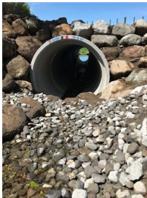
Newly installed culvert
