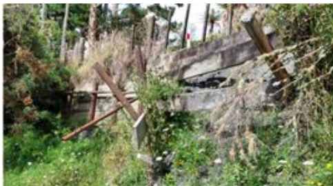
Wall #382: Mangaowata Road
