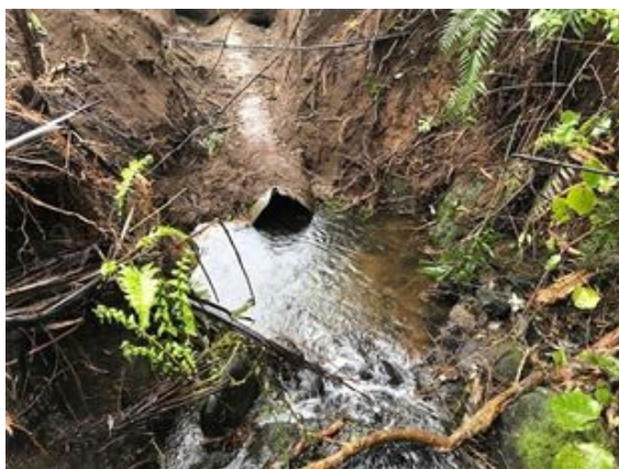
Existing culvert that was removed
