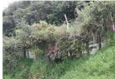
Wall number 227: Mangaehu Road
