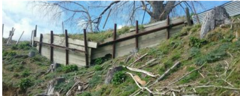
Wall #236: Mangaotuku Road
