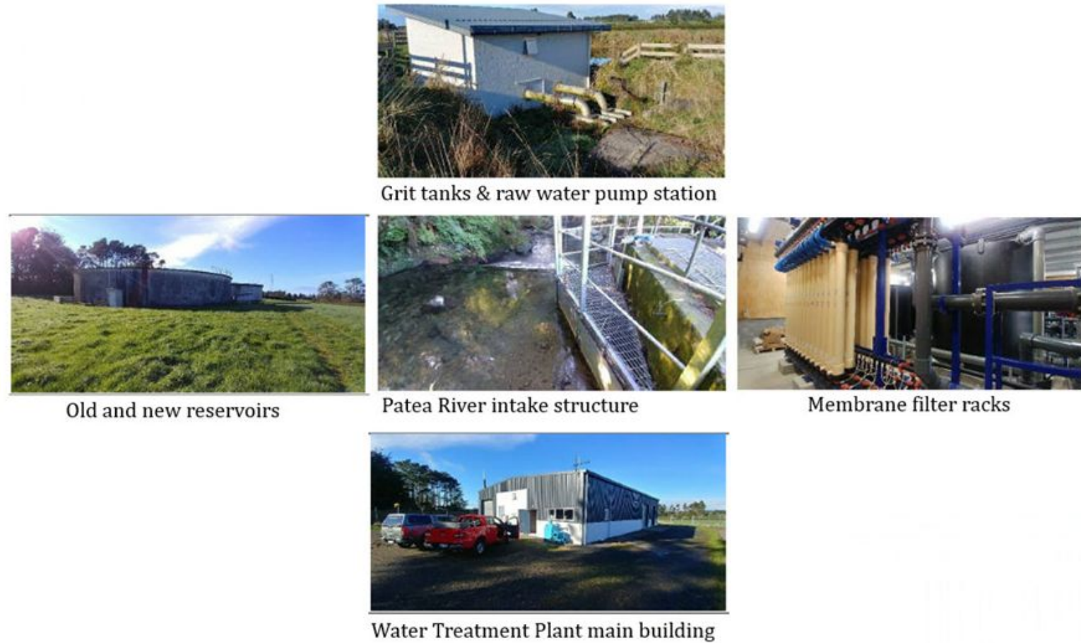
Figure 11 - Stratford Water Treatment Plant Photos
