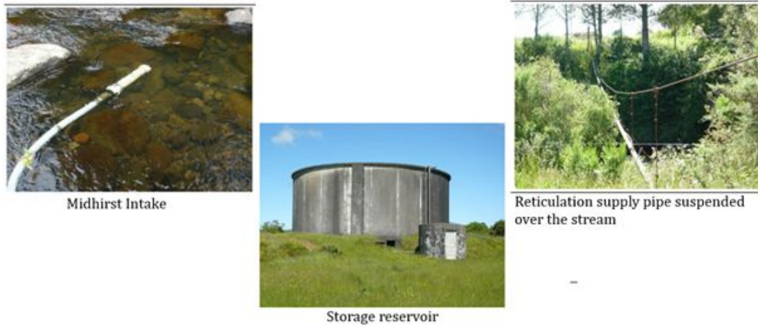
Figure 13 - Midhirst Water Plant Photos
