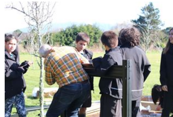
Below: Students at Avon Primary School, a Waste Levy Fund recipient, installing new composting systems for their community garden project.
