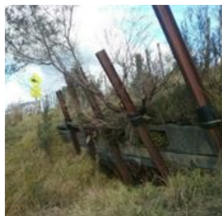
Wall #178: Mangaotuku Road
