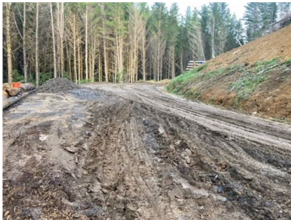
Figure 44 - Photo of Mangaoapa Road
