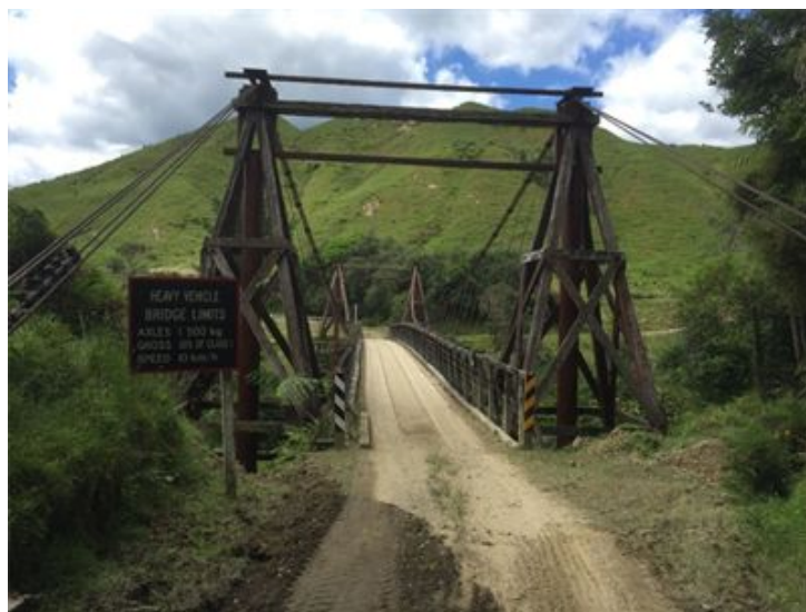
Figure 33 - Lower Kohuratahi Road Bridge
