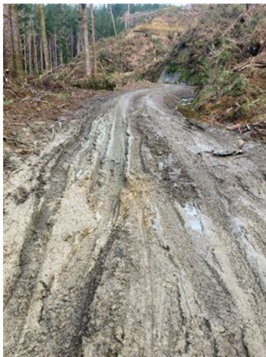
Figure 46 - Photo of Mangaoapa Road
