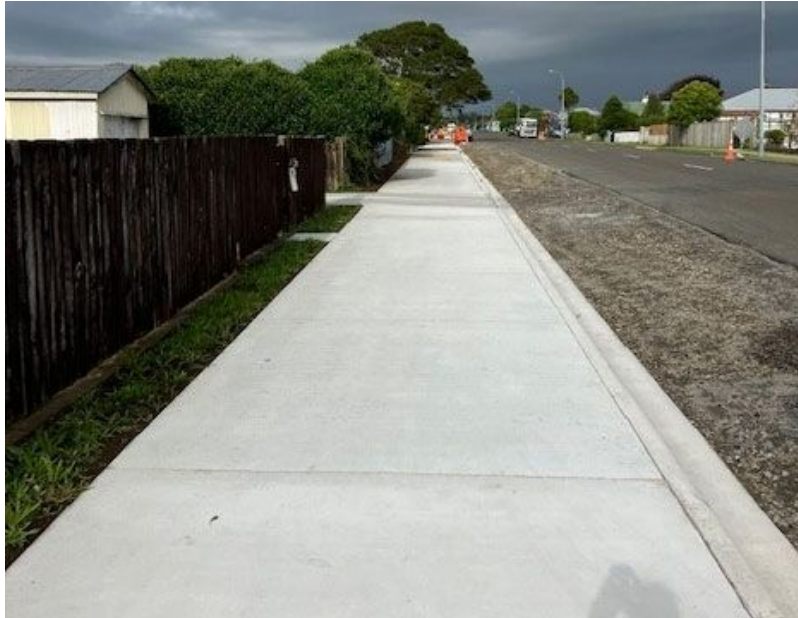
Figure 1: Work progressing on Fenton Street
