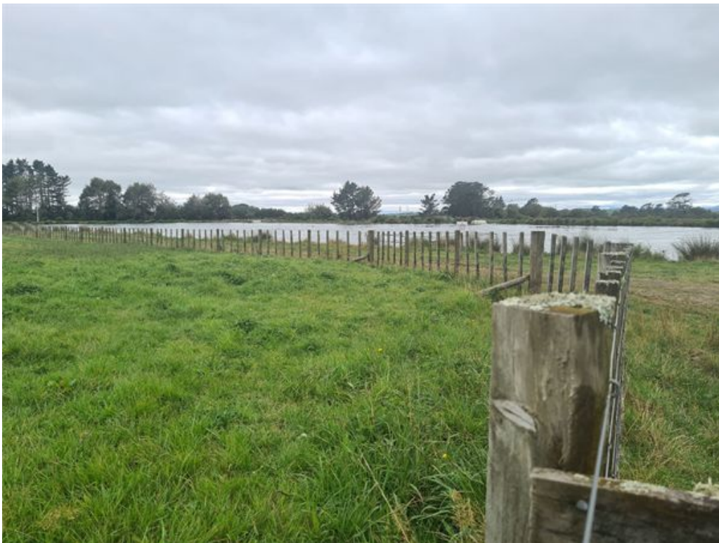
Figure 6: A portion of the current stock fencing around the oxidation pond, there is no electrified wire on the fence.
