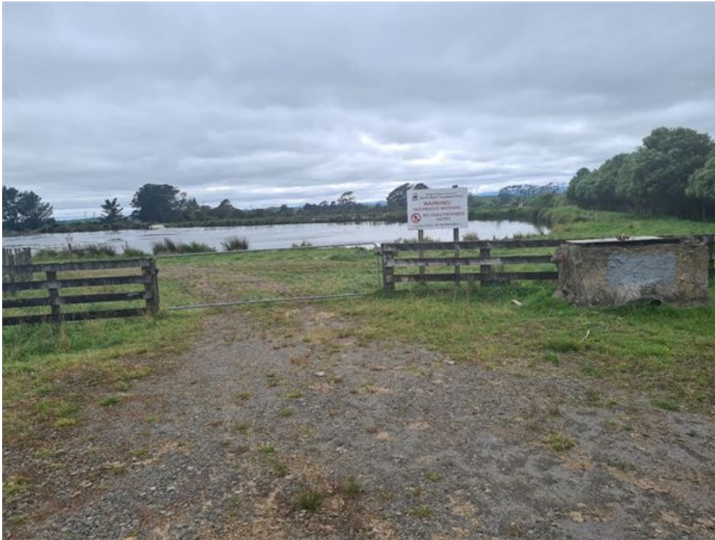
Figure 5: The current access gate to the wastewater oxidation pond, there is no electrified wire on the fence.
