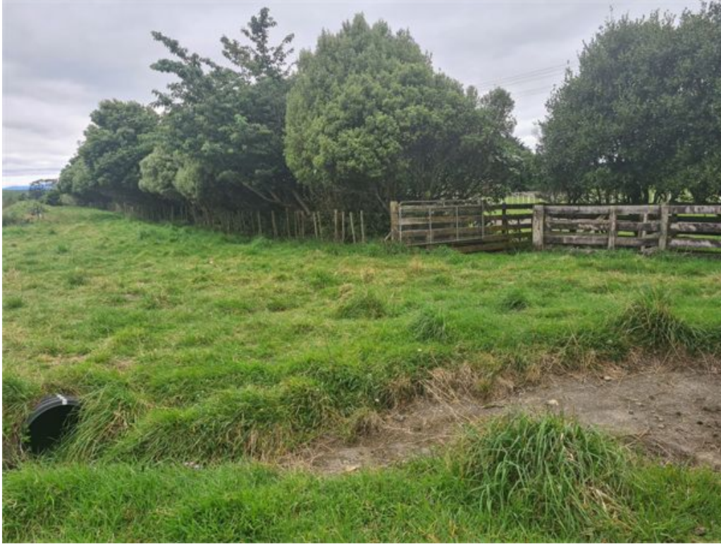
Figure 7: The stock fencing that follows the roadside portion of the wastewater oxidation ponds
