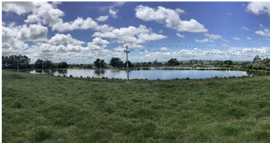
Figure 2: Stratford Wastewater Treatment Ponds
