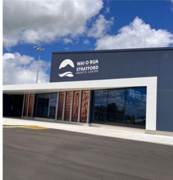
Figure 17: Wai o Rua – Stratford Aquatic Centre
