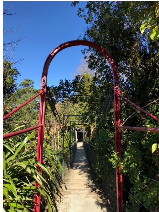
Figure 8: King Edward Park swing bridge.
