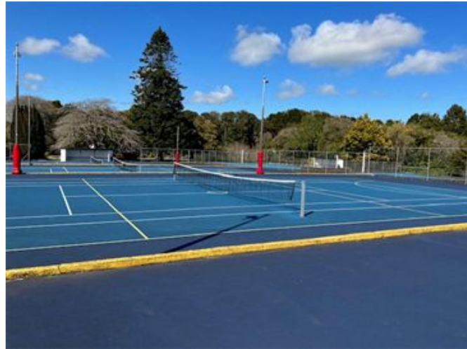
Figure 26: Netball & Tennis Courts
