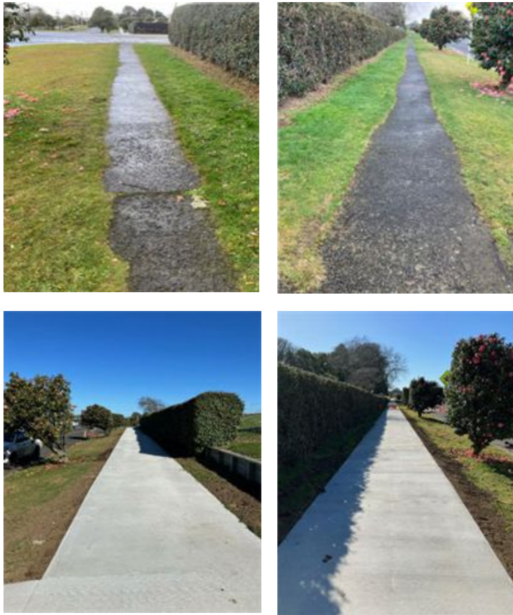
Figure 3: The replacement footpath on Cordelia
