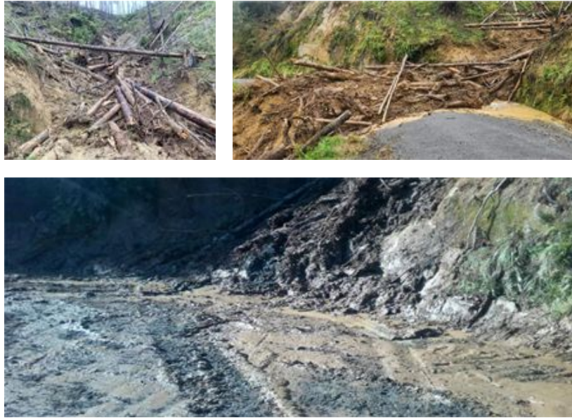
Figure 2: Landslip on Mangaehu Road
