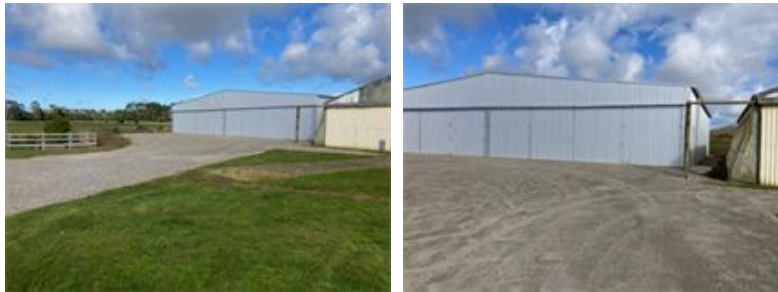
Figure 8: Completion photos of the Aero Clubs new hangar - August 2023
