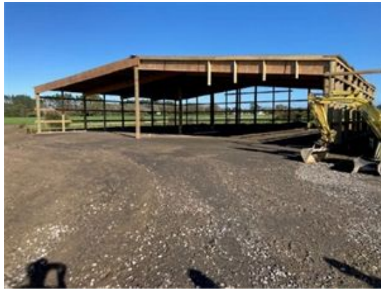
Figure 6: New Aero Club hangar construction in progress
