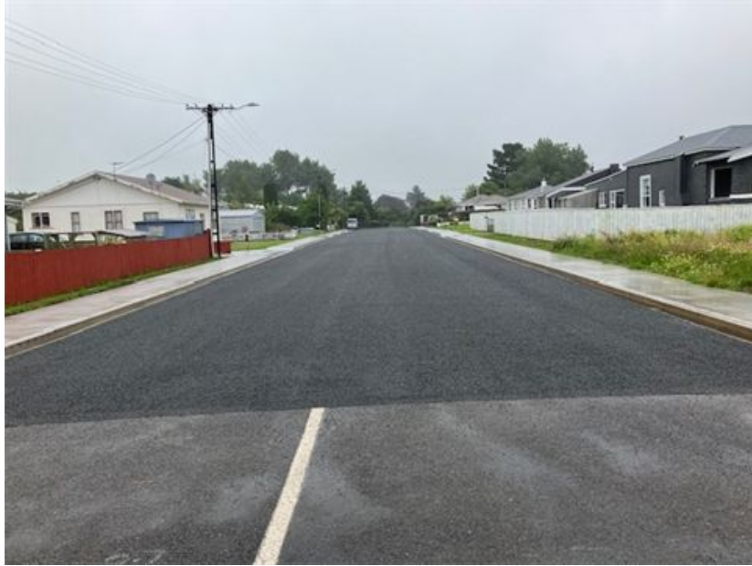
Figure 4: Completed work on Elsinore Street
