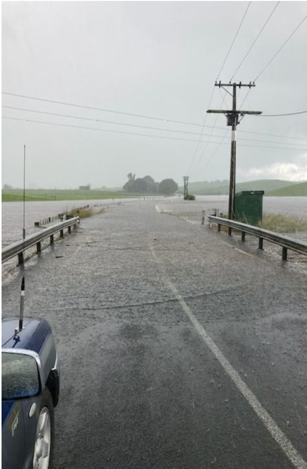
Figure 1: Flooding on Cheal Road
