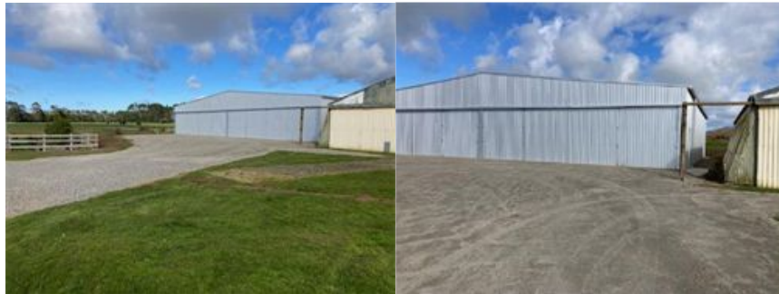
Figure 2: Completion Photos of the Aero Club new Hagar
