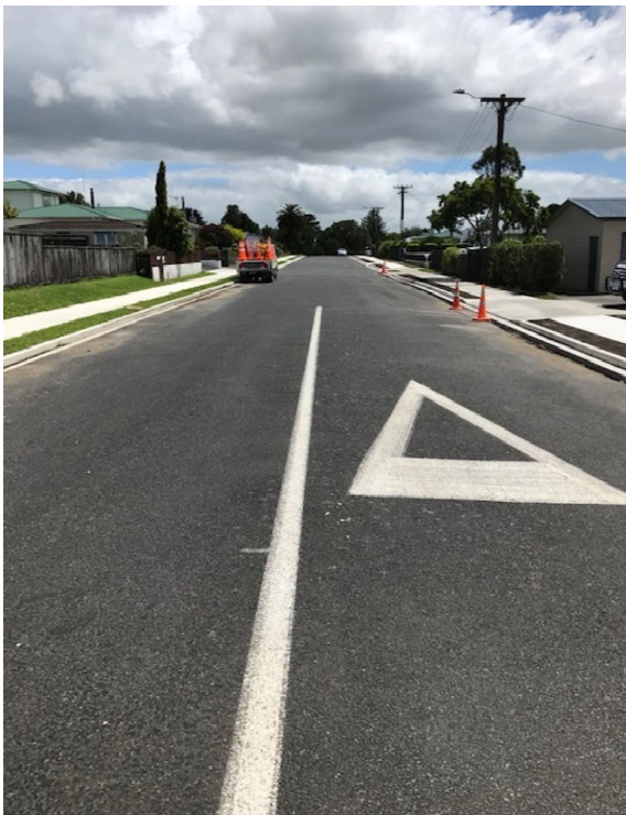
Figure 5: Fabian Street with new kerb, channel, and footpath
