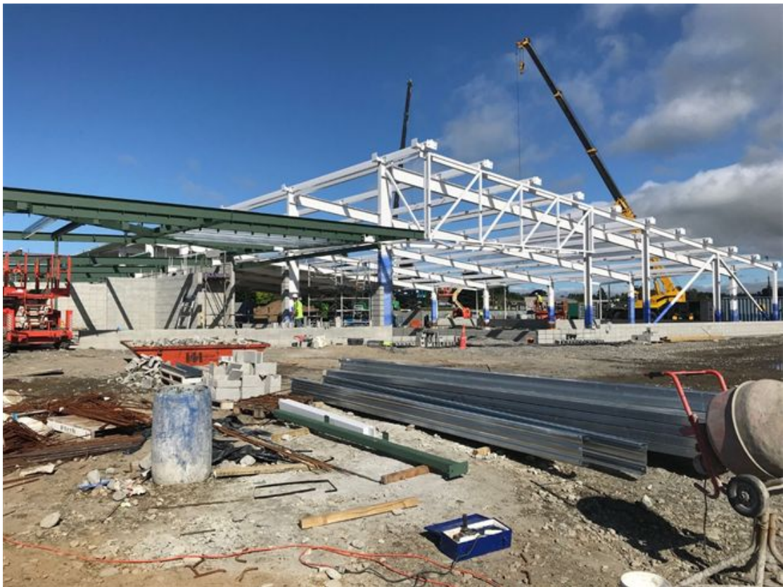
Figure 13: New aquatic centre portal steelwork almost completed.
