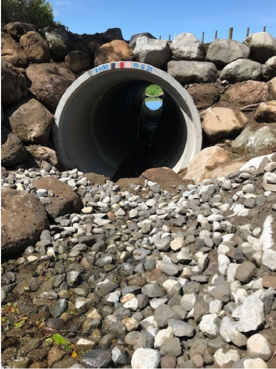
Figure 4: The replacement culvert installed under Manaia Road at Hollard Gardens
