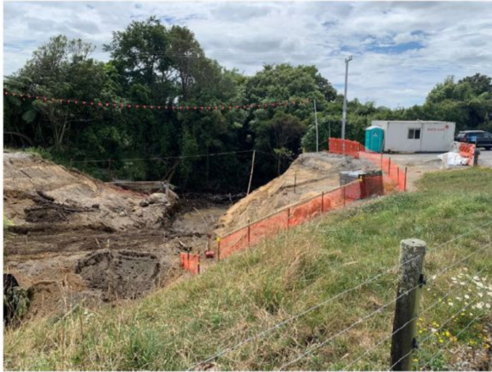
Figure 1: Excavation to expose the existing steel culvert
