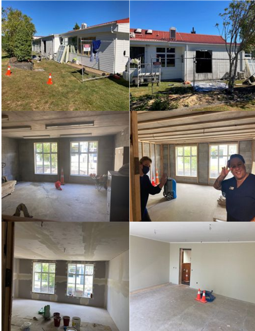
Figure 6: Safe Conversion Progress photos
