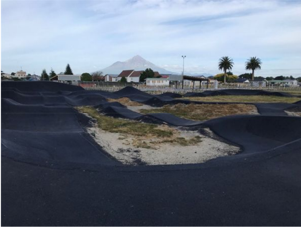
Figure 9: The Children's Bike Park pump track nearing completion
