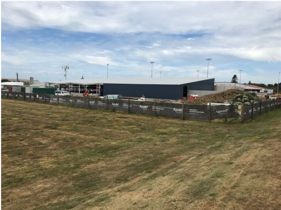
Figure 8: New aquatic centre external cladding well underway.
