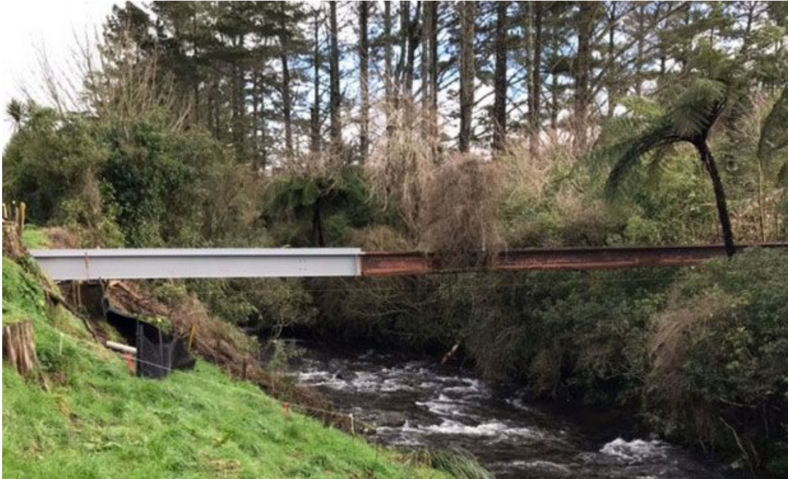
Figure 4: New pipe-bridge welded to old pipe-bridge during replacement installation
