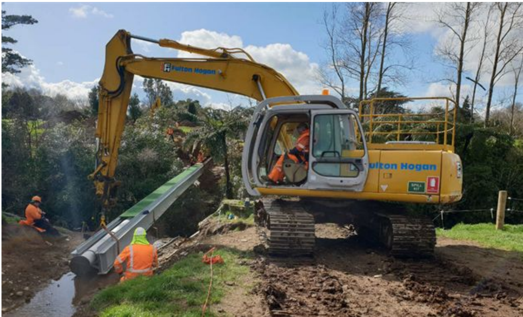
Figure 5: New pipe-bridge installed over the Patea River.
