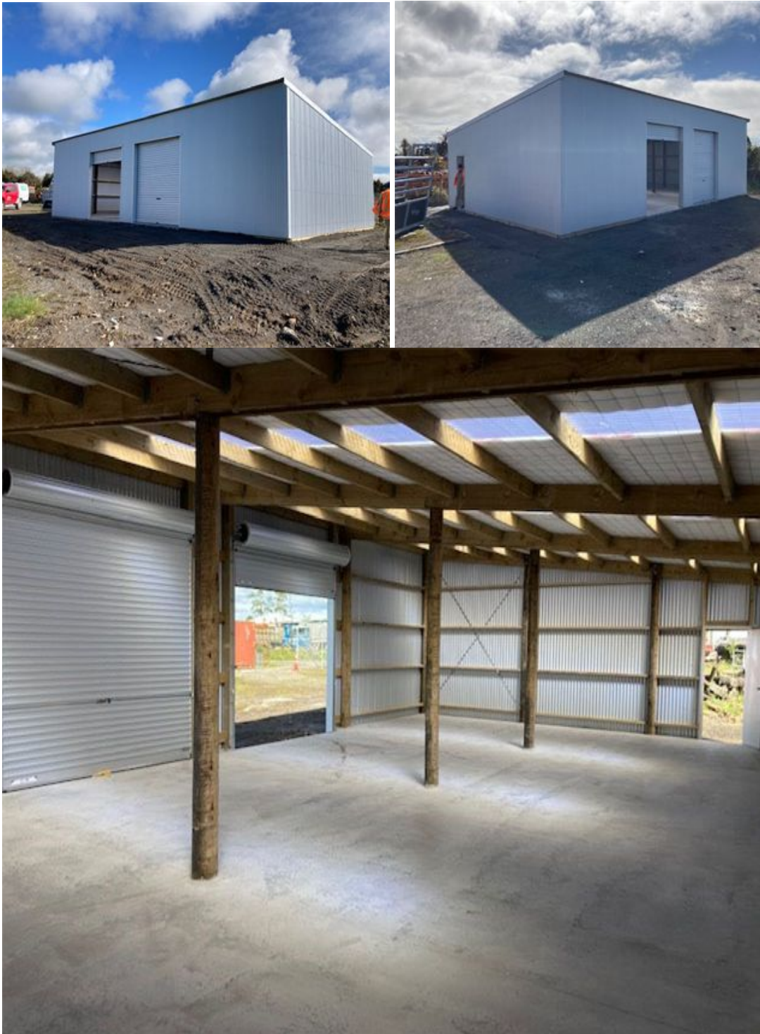
Figure 11: Storage Shed Construction Progress Photos
