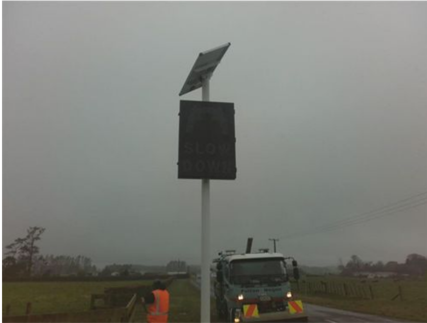
Figure 3: Electronic warning sign on Beaconsfield Road
