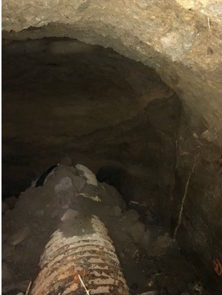
Figure 8: Manaia Road Culvert - Hollard Garden., Culvert replaced and road re-constructed. Cost = $303,000
