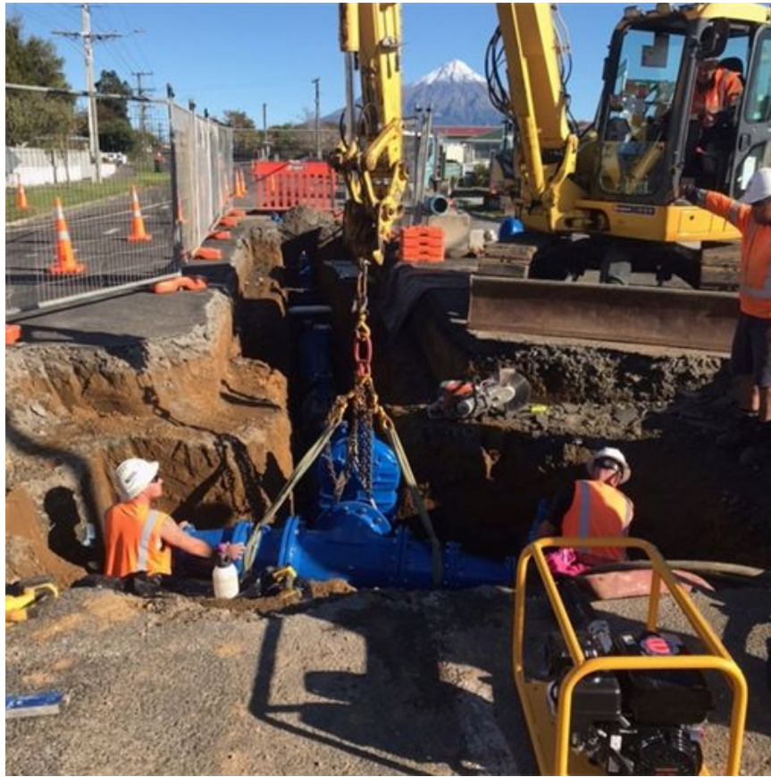
Figure 5: Trunk-main valve installation at Brecon/Pembroke Road intersection
