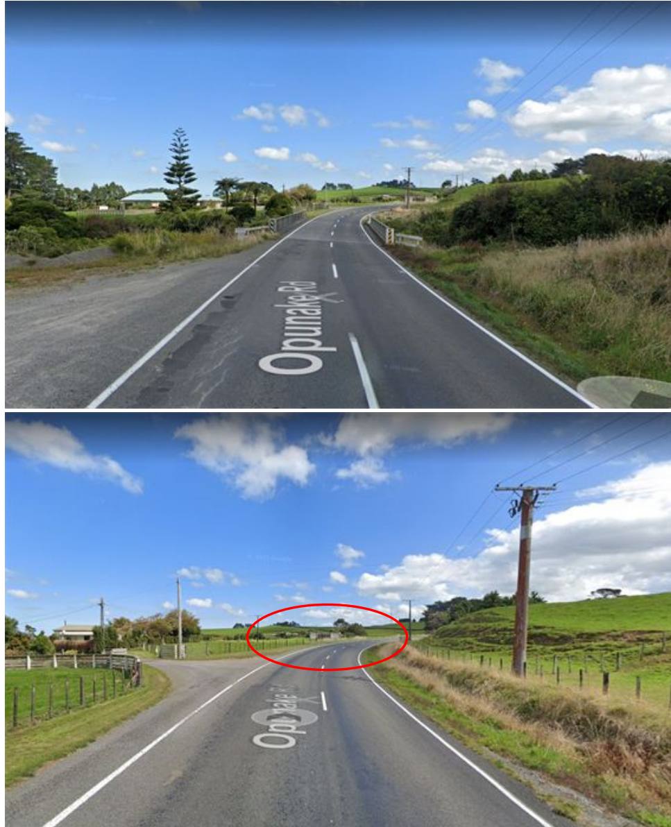
From Stratford towards Mahoe with Bridge 110 showing the blind corner which can be slippery when wet and has no warning signs. There have been many crashes into the fence in the area circled
