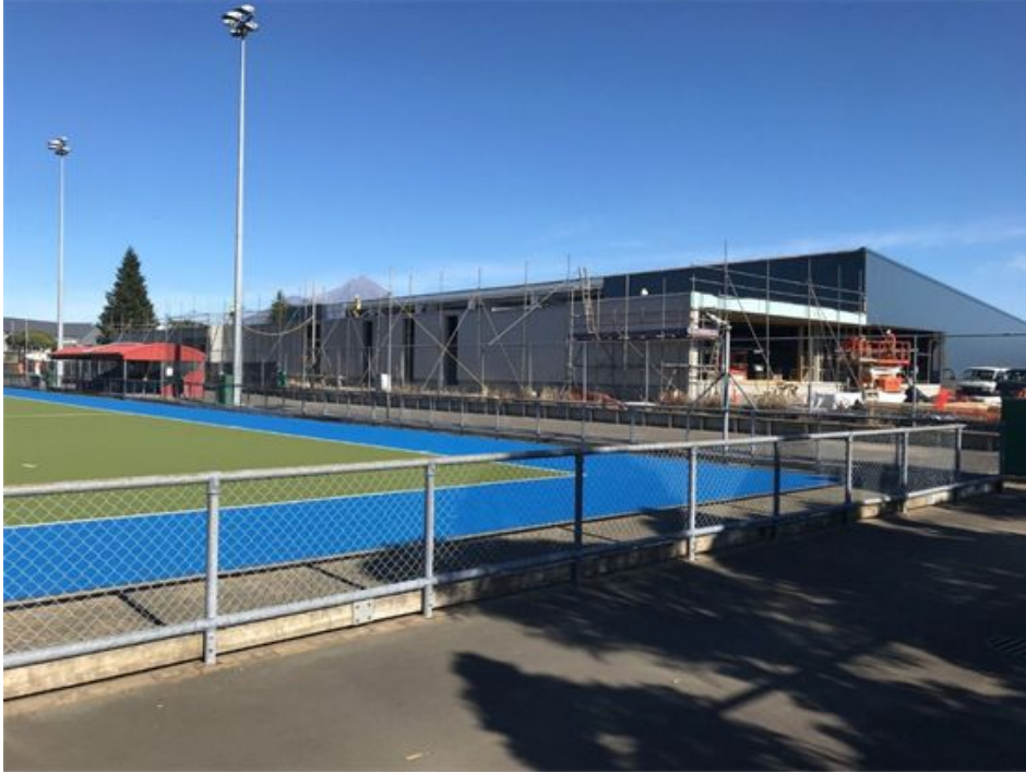
Figure 13: Aquatic Centre external cladding complete
