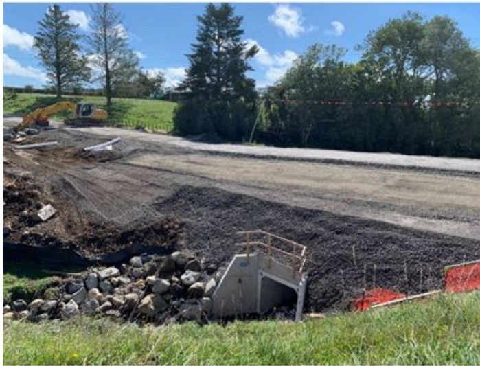
Figure 4: Backfill material up to 200mm of the finished road level
