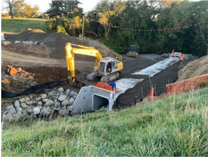
Figure 3: Backfill material being placed over the culvert
