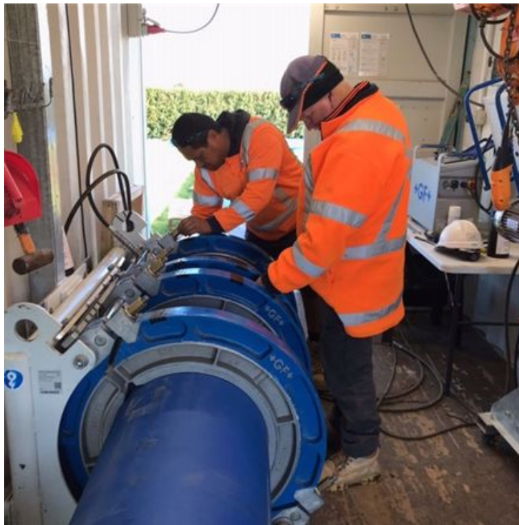
Figure 6: Stage 3, 2nd Trunkmain Project
