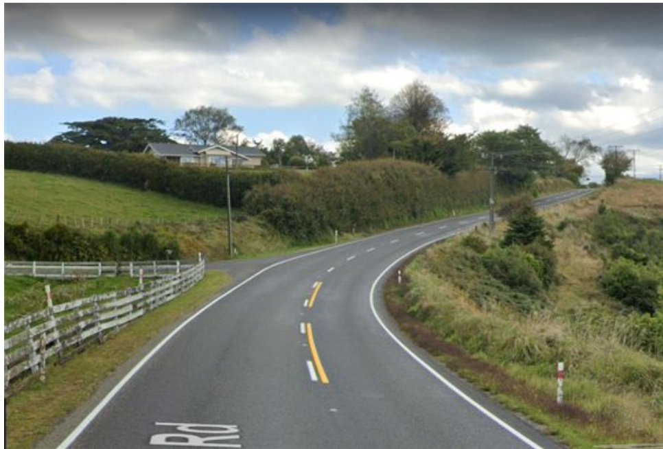
From Stratford towards Cardiff - a series of blind corners from about 255 Opunake Road with no warning signs. This can be deceptive, particularly at night or in fog.
