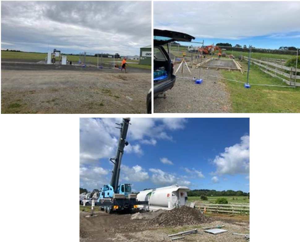
Figure 3: Progress photos of the Jet A1 Fuel holding tank being installed.
