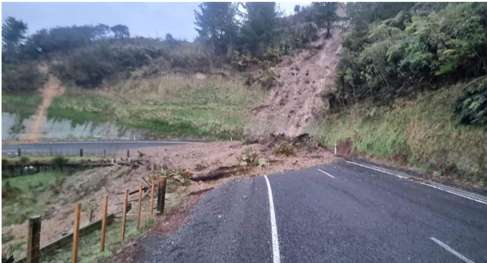
Figure 1: Slip on Mangaotuku Road following heavy rainfall event on Sunday 29 August
