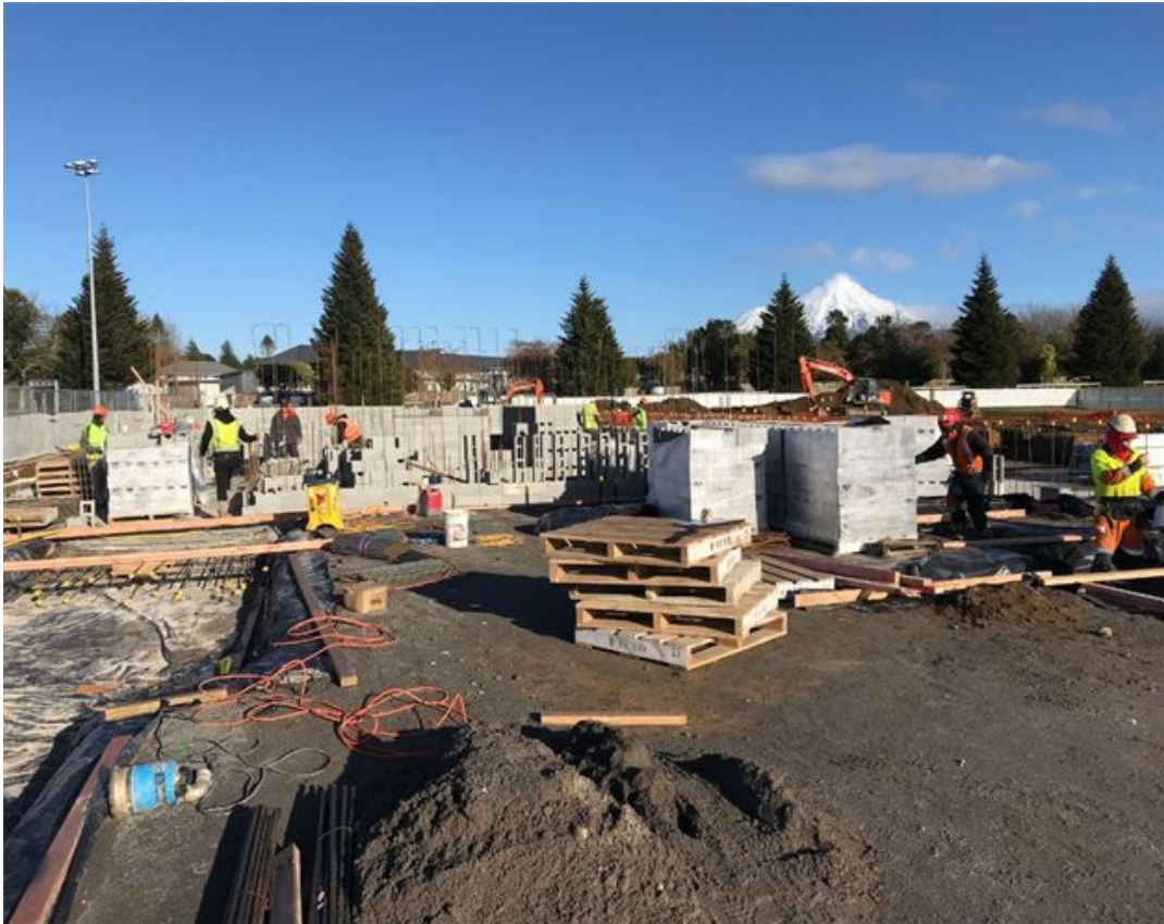
Figure 6: New aquatic centre dryside blockwork well underway pre-Covid lockdown.
