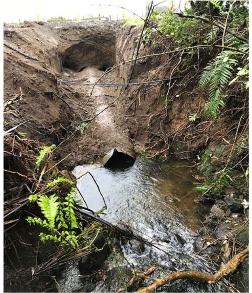
Figure 2 – The roof of the cavity removed exposing the steel culvert
