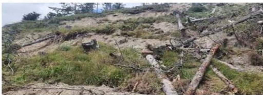
Figure 3: Slip on Whitianga Road which was cleared in January.
