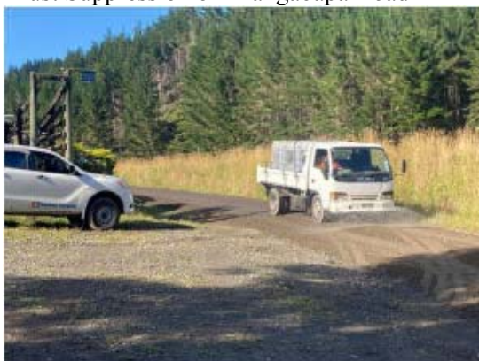
Figure 1 – Dust Suppressant being sprayed on Mangaoapa Rd.
