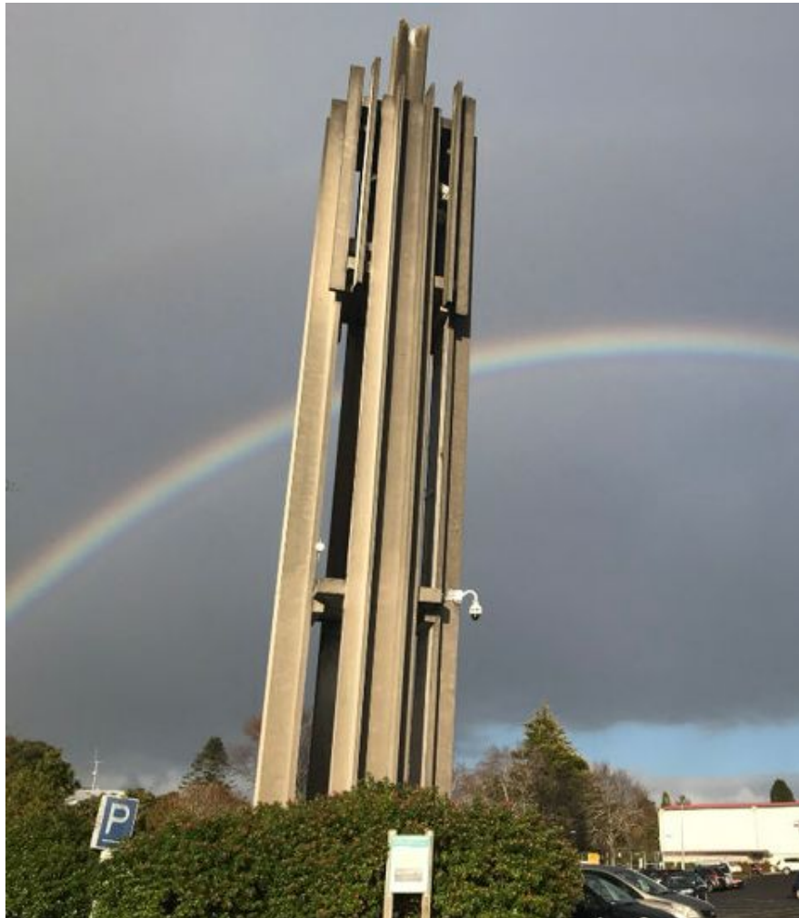
Figure 35 - Bell Tower, Miranda Street, Stratford
