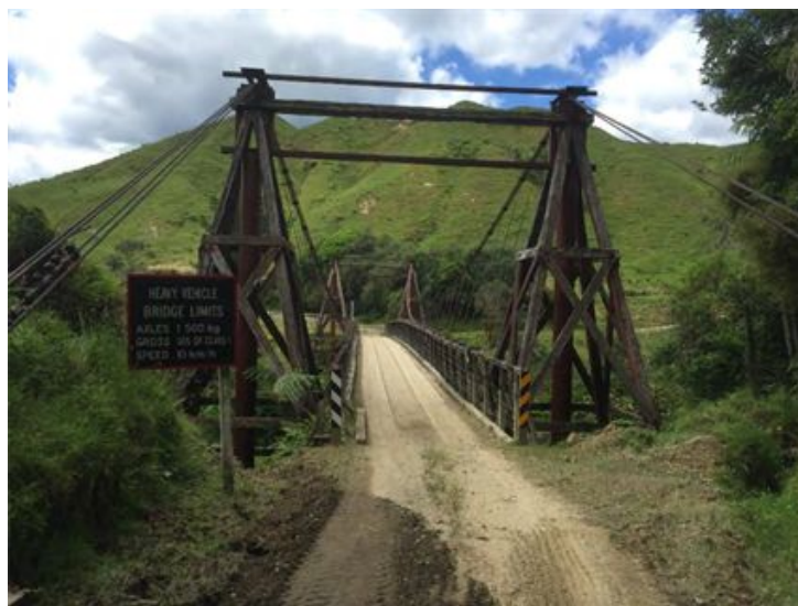
Figure 38 - Lower Kohuratahi Road Bridge
