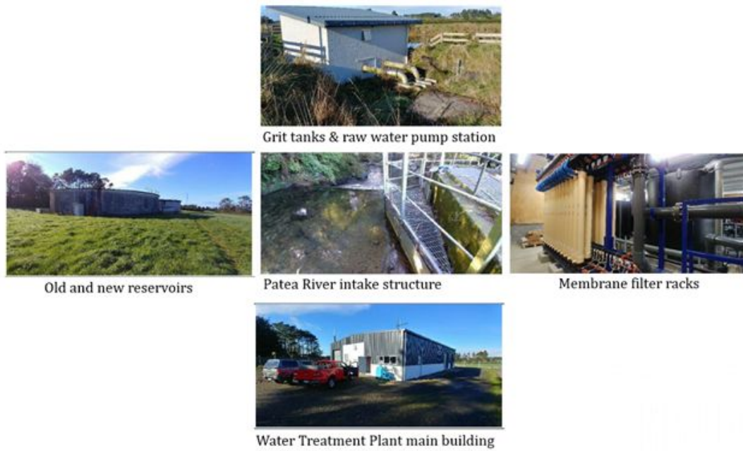
Figure 9 - Stratford Water Treatment Plant Photos
