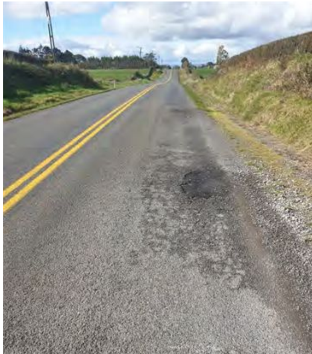
Figure 52 - Photo of Opunake Road
