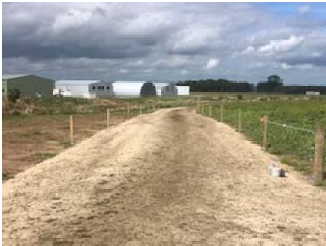
Farm Race completed with Fencing
