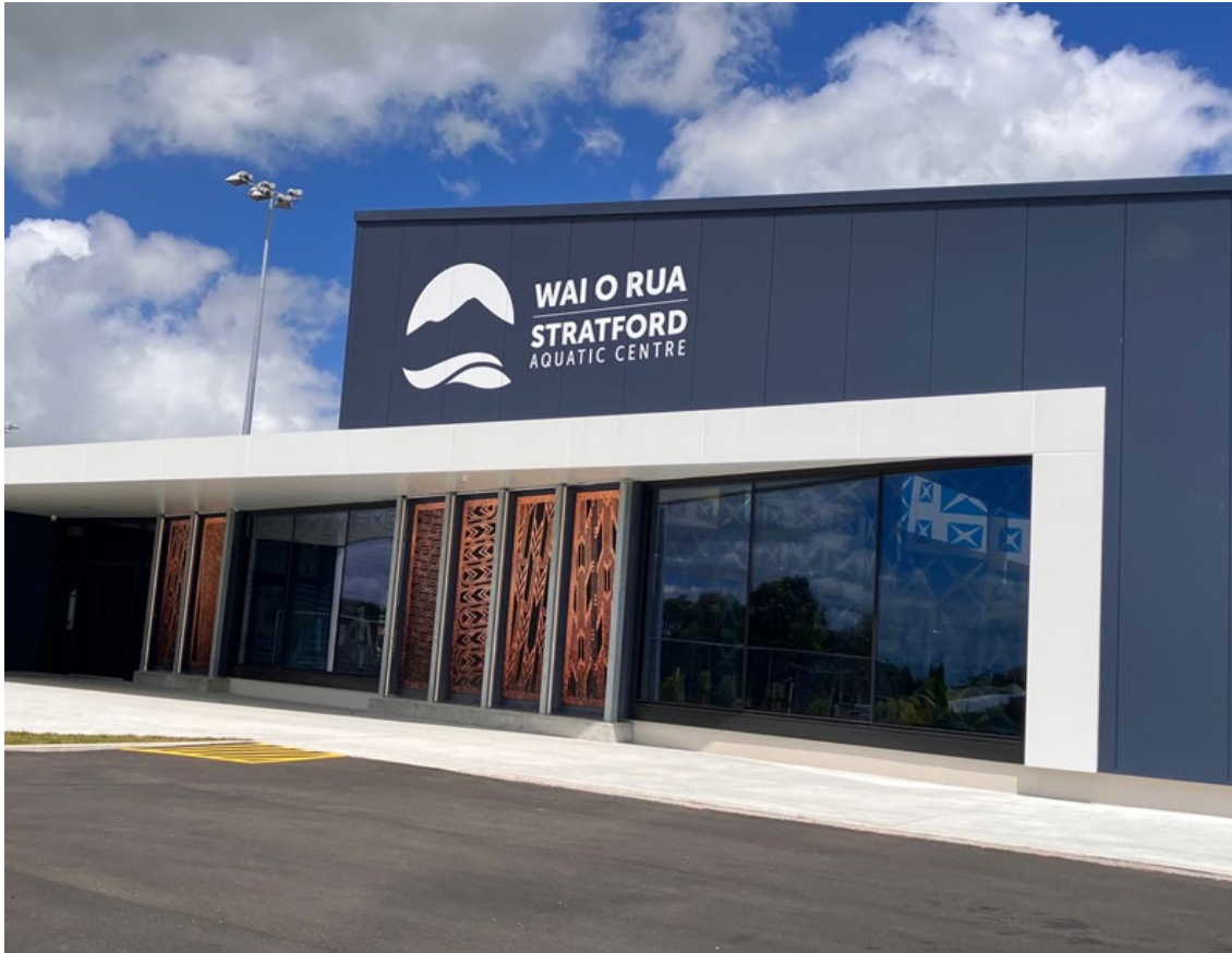
Figure 17: Wai o Rua – Stratford Aquatic Centre
