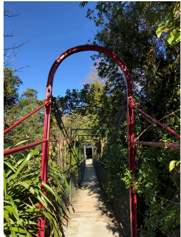
Figure 8: King Edward Park swing bridge.
