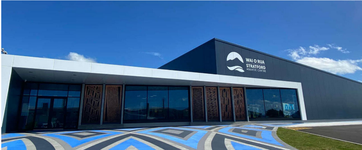
Figure 9 – Wai o Rua -Stratford Aquatic Centre
