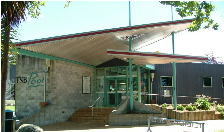
Figure 34 TSB Pool Complex
