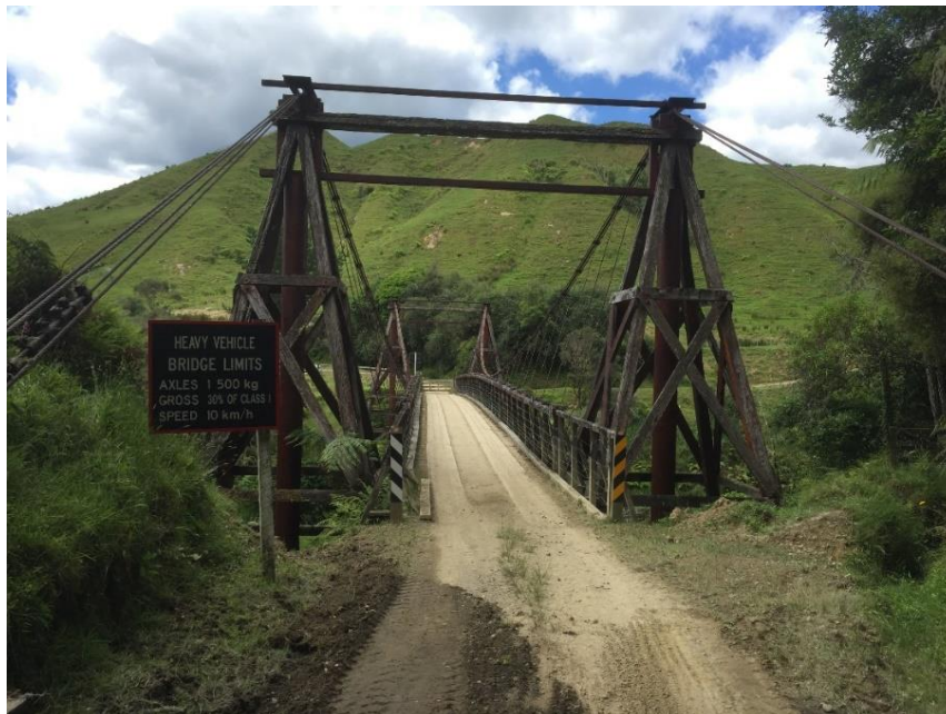
Figure 38 - Lower Kohuratahi Road Bridge
