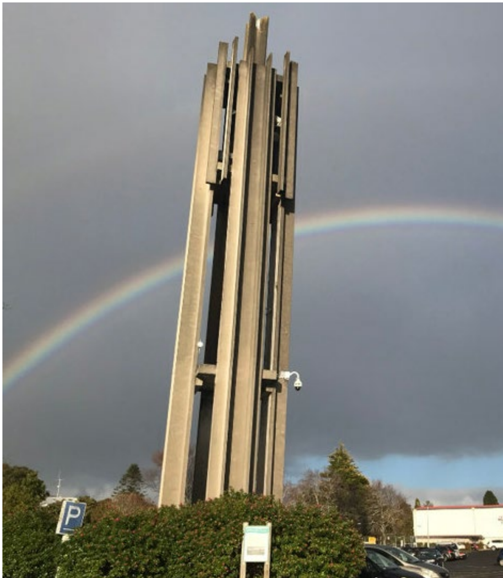
Figure 35 - Bell Tower, Miranda Street, Stratford
