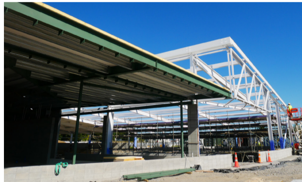
Roofing on the new Aquatic Centre is making good progress.
