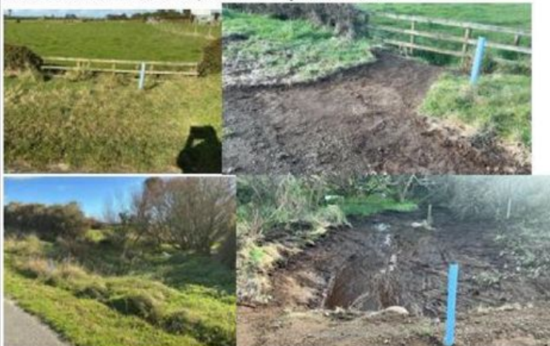
Figure 4: Low shoulder and drainage works
