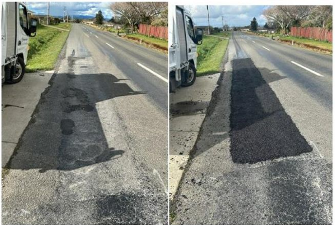
Figure 3: Grading and level depression
