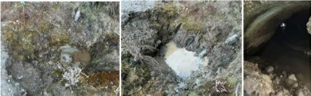
Figure 1: Bridge and Drainage cleaning
