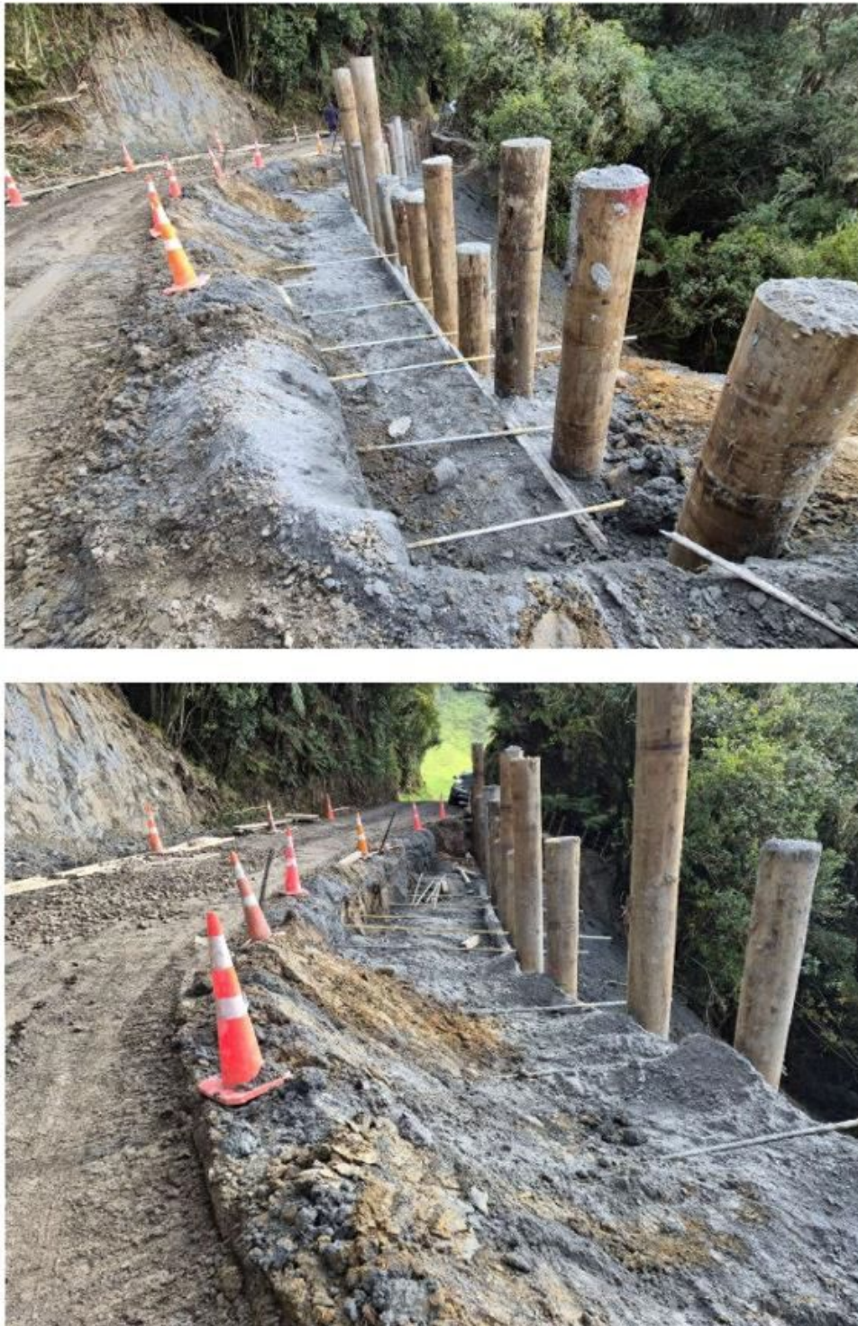
Figure 6: A new retaining wall under construction on Junction Road
