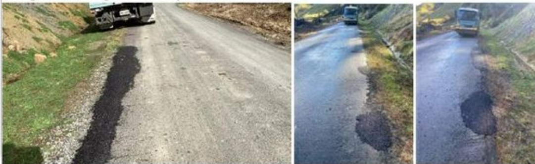
Figure 2: Culvert cleaning, footpath repairs, edge breaks
