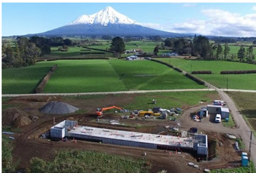
Figure 6: Grit Tank – Ongoing Construction
