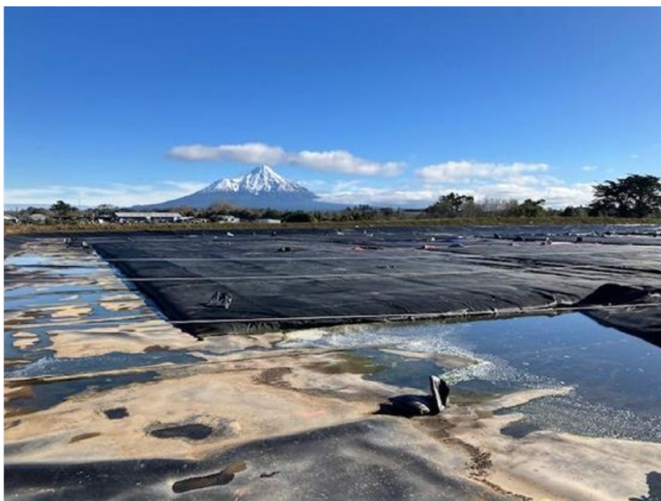
Figure 7: Geotextile Bag Filling Ongoing During Dredging Operations
