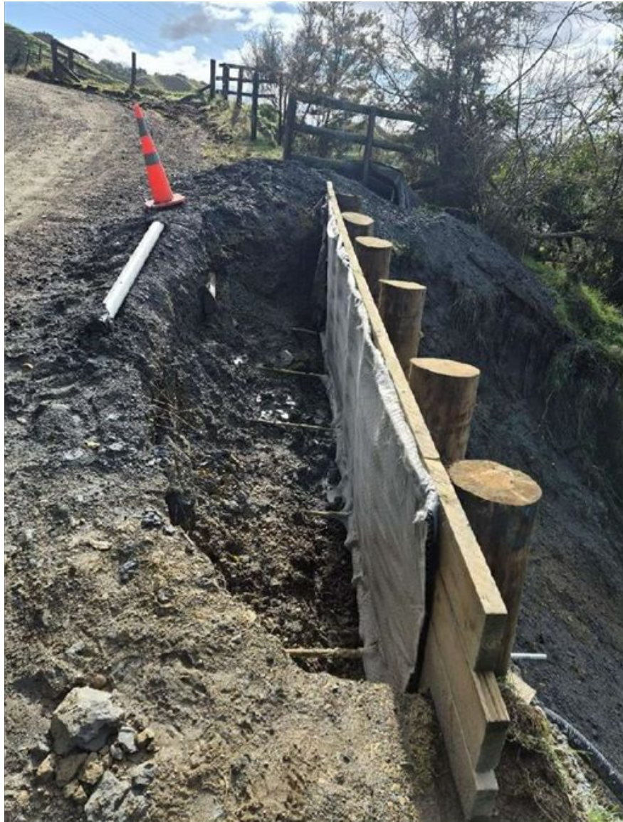
Figure 4: A new retaining wall under construction on Whitianga Road
