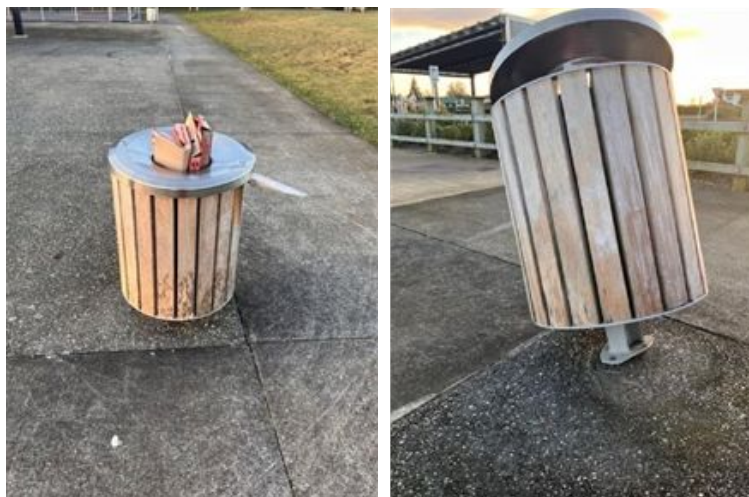
Figure 20: Vandalised Rubbish Bins at Victoria Park
