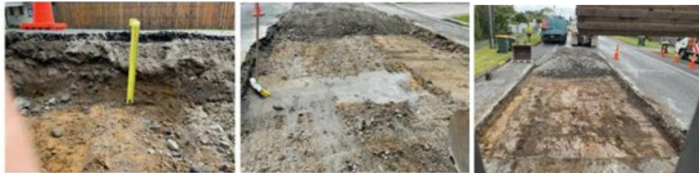
Figure 2: Pavement repairs on Celia Street.
