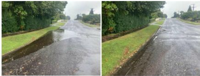
Figure 3: Brecon Road Flooding.
