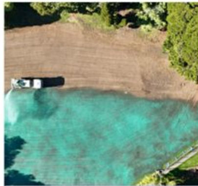
The old TSB Pool Complex was demolished and the area returned to a green space.
