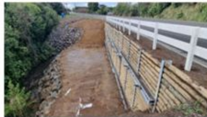
New retaining wall completed on Opunake Road
