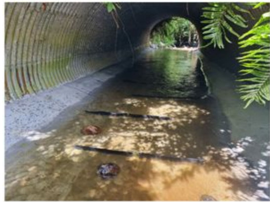
Figure 2: The completed concrete lining with rubber baffles for the fish passage
