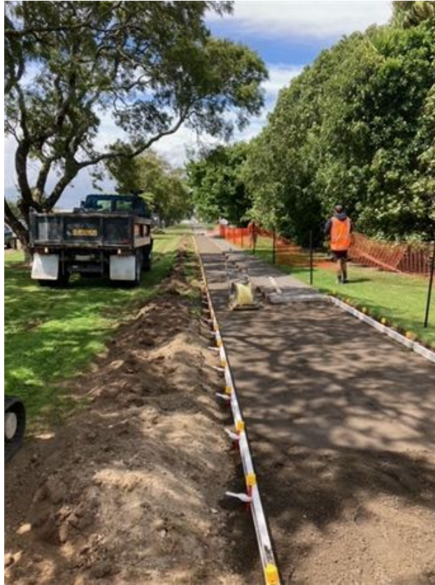
Figure 4: Widening of the footpath on Regan Street.
