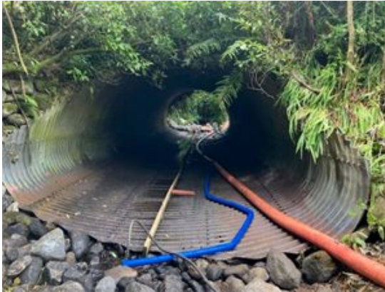
Figure 1: De-watering of the Culvert under Pembroke Road West.
