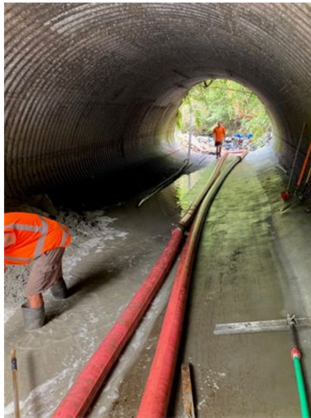
Figure 3: Concrete lining being poured.
