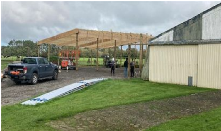
Figure 6: New Aero Club hangar construction in progress
