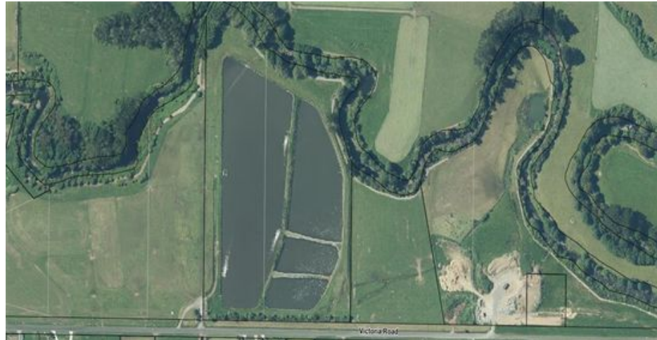
Figure 1: An aerial view of the Wastewater Treatment Ponds
