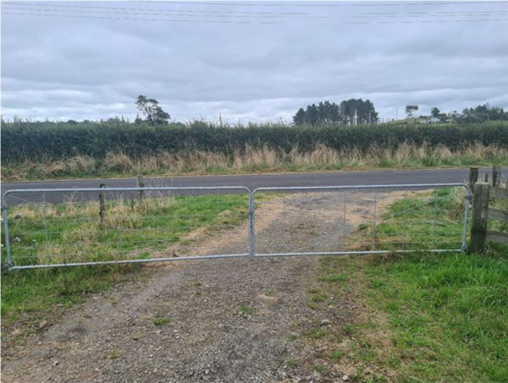
Figure 4: The other current outer gate onto the wastewater oxidation pond property, one side lacks electrified wire.
