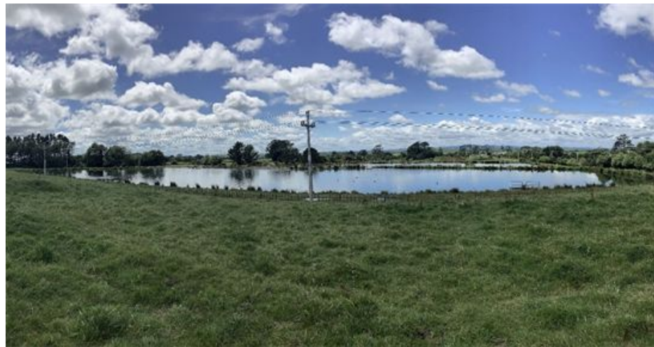
Figure 2: Stratford Wastewater Treatment Ponds
