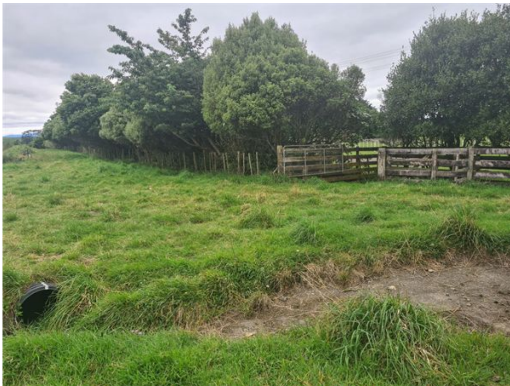
Figure 7: The stock fencing that follows the roadside portion of the wastewater oxidation ponds
