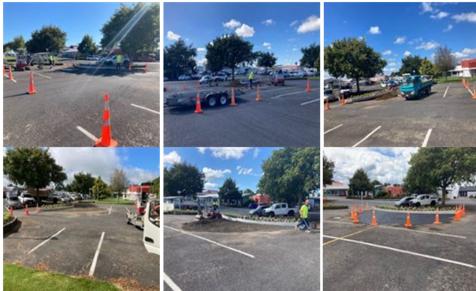
Figure 5: Progress and completion photos of the War Memorial carpark reinstatement
