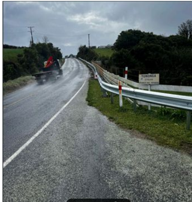
Figure 1: The Armco roadside barrier installation on Opunake Road
