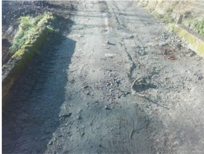
Figure 2: Before repairs - Concrete bridge on Puniwhakau Road
