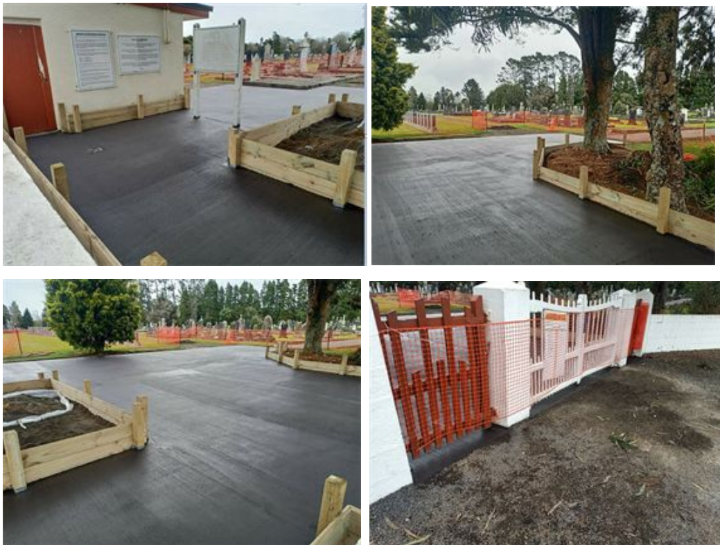
Figure 16: Progress photos of Kopuatama Cemetery Entrance Upgrade
