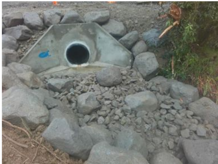
Figure 3: After repairs - The outlet of the culvert pipe on Puniwhakau Road
