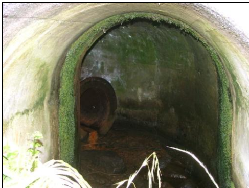
Inner view of pipes and culverts which originally would have fed water wheel
