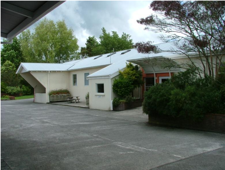
Stratford Dairy Company
