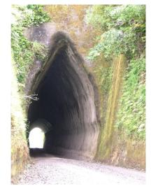
the concrete on the floor of the tunnel and had a worker shovel it onto a platform and plaster it onto the roof with his shovel. By 1958, the south end of the tunnel was gunited (the concrete was coated) and was therefore declared safe.
