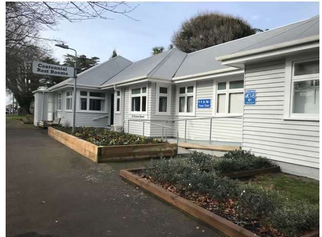
Figure 22: Centennial Rest Room & Front Gardens
