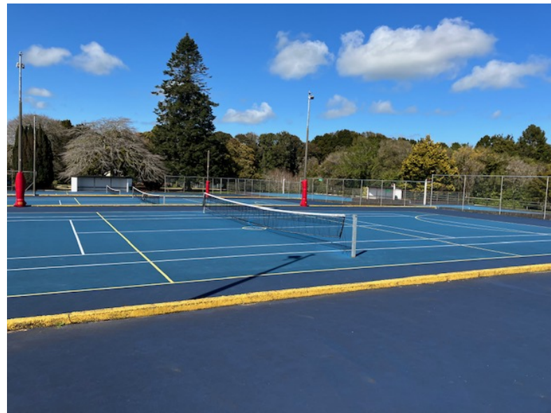
Figure 26: Netball & Tennis Courts
