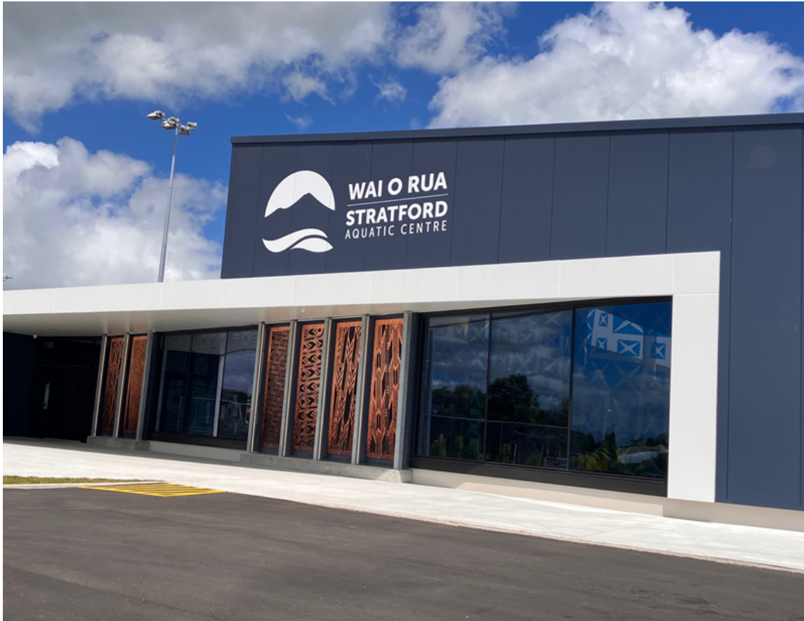
Figure 17: Wai o Rua – Stratford Aquatic Centre
