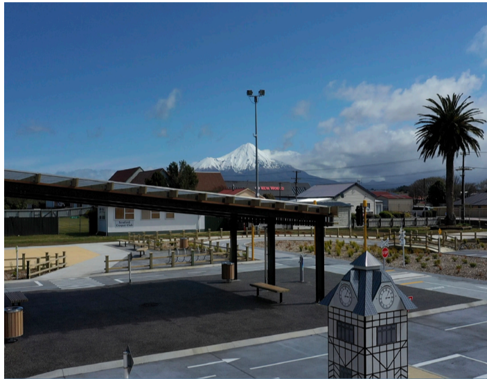
Completion of the new children's bike park and half basketball court.
