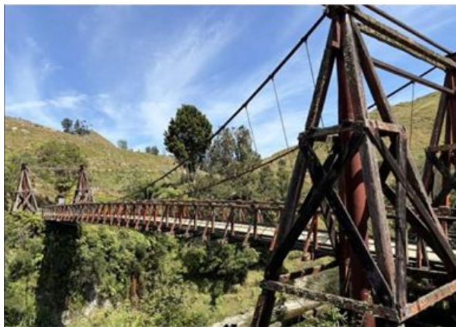
Figure 3: Lower Kohuratahi Bridge #2 as seen from the eastern side of the Tangarakau River
