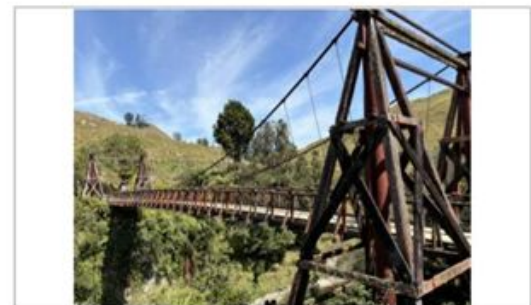
Bridge - east view
