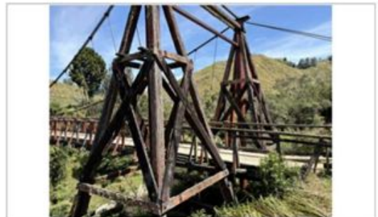
Columns - east end
