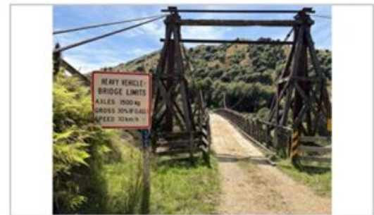
Western approach and old sign
