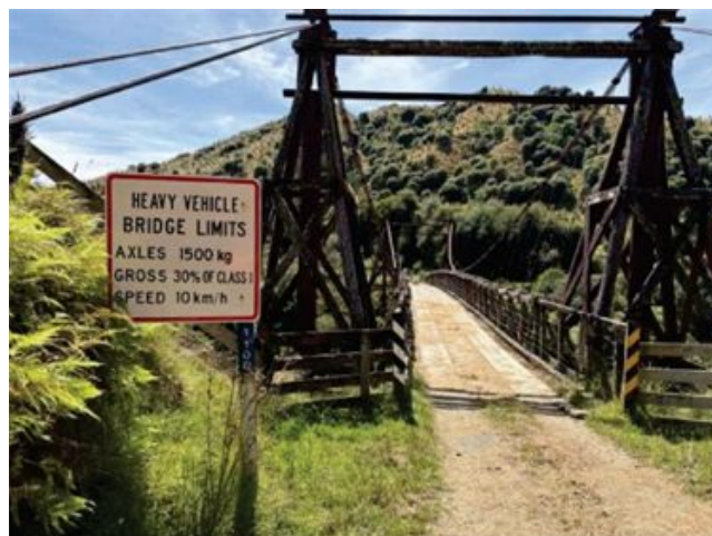
Figure 4: Western approach of the Lower Kohuratahi Bridge #2 showing the current signage.
