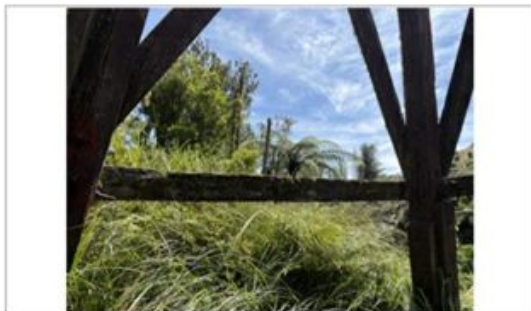
Timber supporting column - west end
