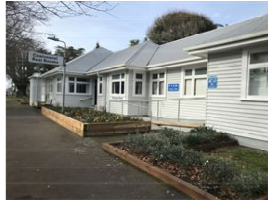
Figure 23: Centennial Rest Room & Front Gardens
