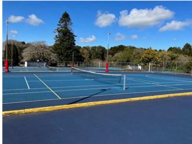
Figure 27: Netball & Tennis Courts
