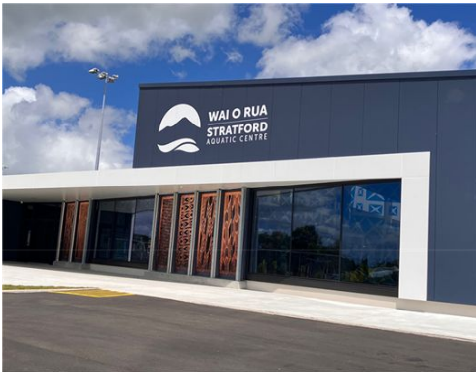
Figure 18: Wai o Rua – Stratford Aquatic Centre
