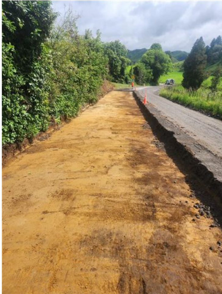
Figure 5: Pavement Repairs to Brewer Road
