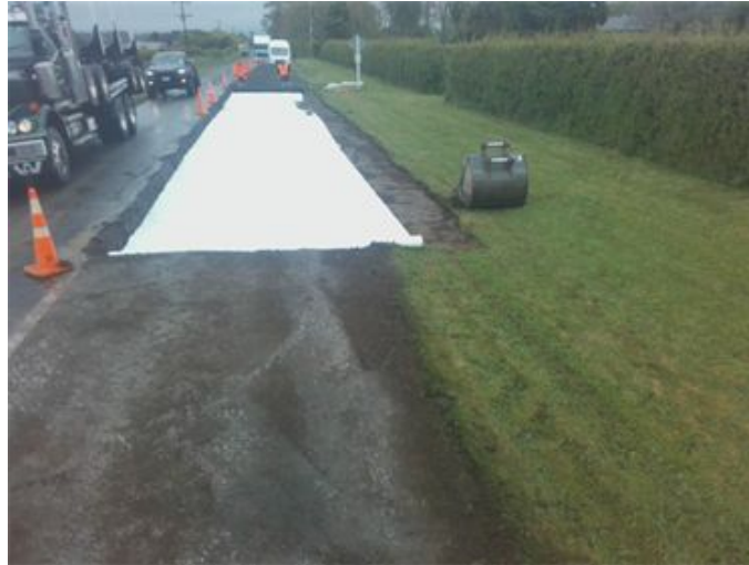
Figure 2: Pavement repairs to Beaconsfield Road.
