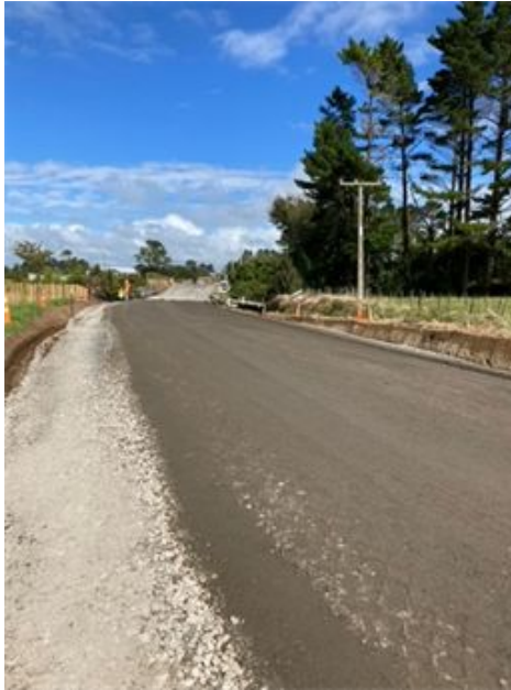
Figure 2: Cardiff Road approaching the Patea River bridge
