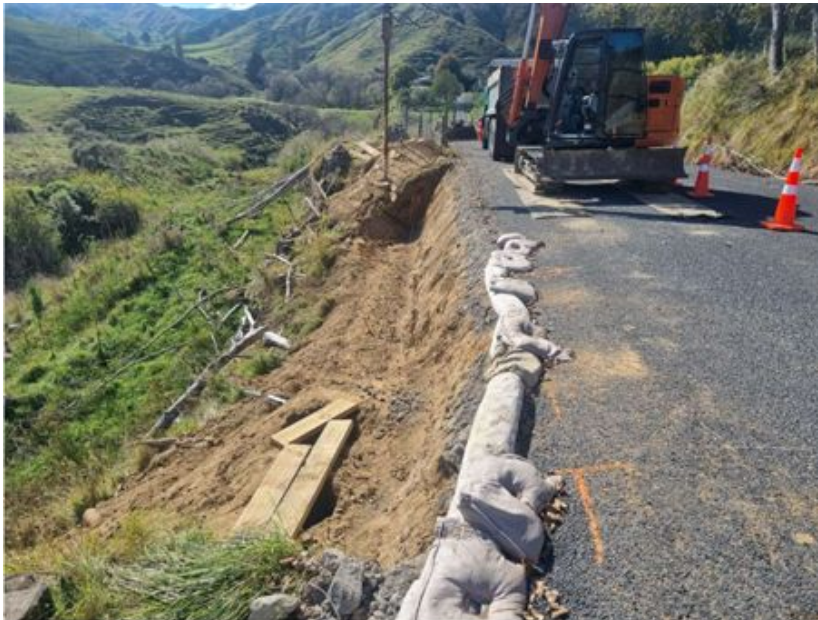
Figure 3: Mangaotuku Rd Retaining Wall RP5.0 - Holes drilled for the steel columns.
