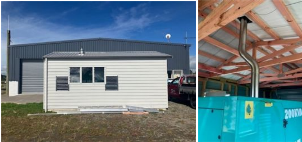
Figure 4: Exterior and interior ventilation installed at the WTP.
