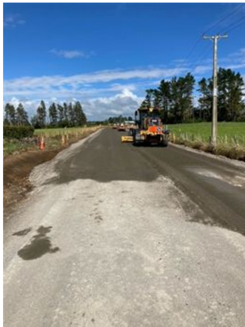
Figure 1: Grading and rolling the AP65 structural metal on Cardiff Road
