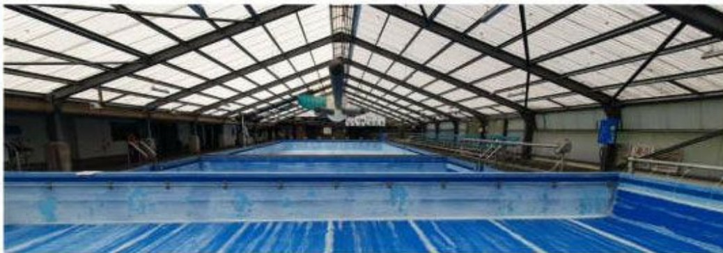
Figure 1: Cold-formed steel portal frame structure
