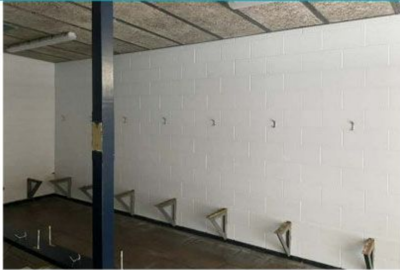
Figure 4: Internal reinforced concrete block wall in annexes
