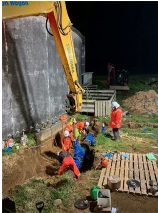
Figure 1: New Trunk Main Tie-in.
