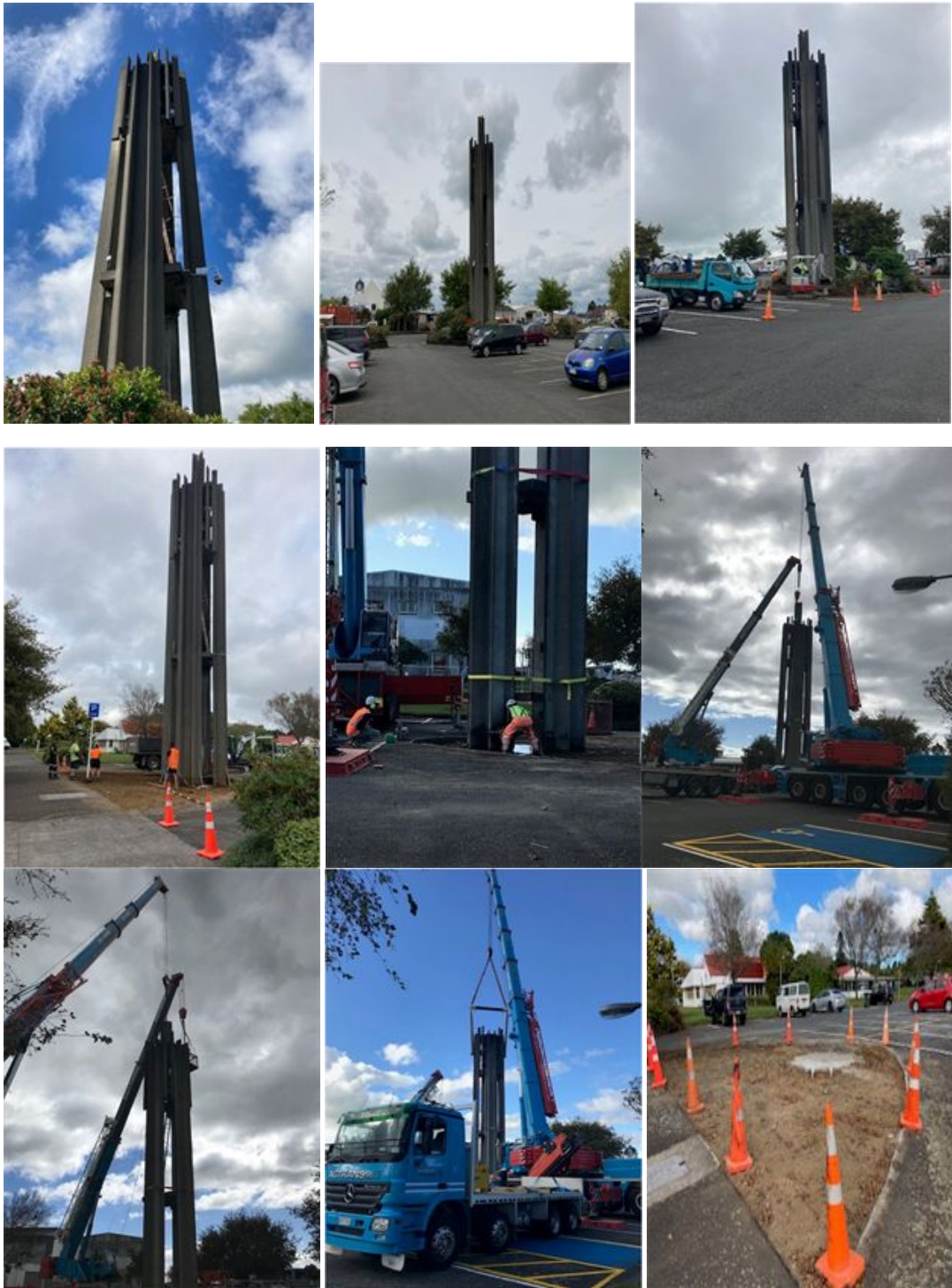
Figure 12: Bell Tower demolition photos.
