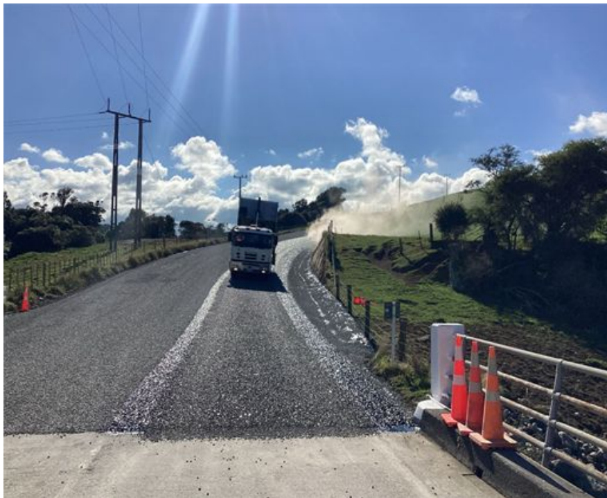
Figure 4: Sealing of Palmer Road including the roadside drain.
