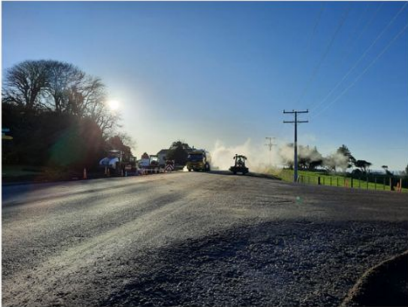
Figure 7: Opunake Road / Palmer Road – Final preparations before sealing
