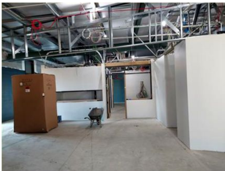
Figure 17: Progress on Reception
