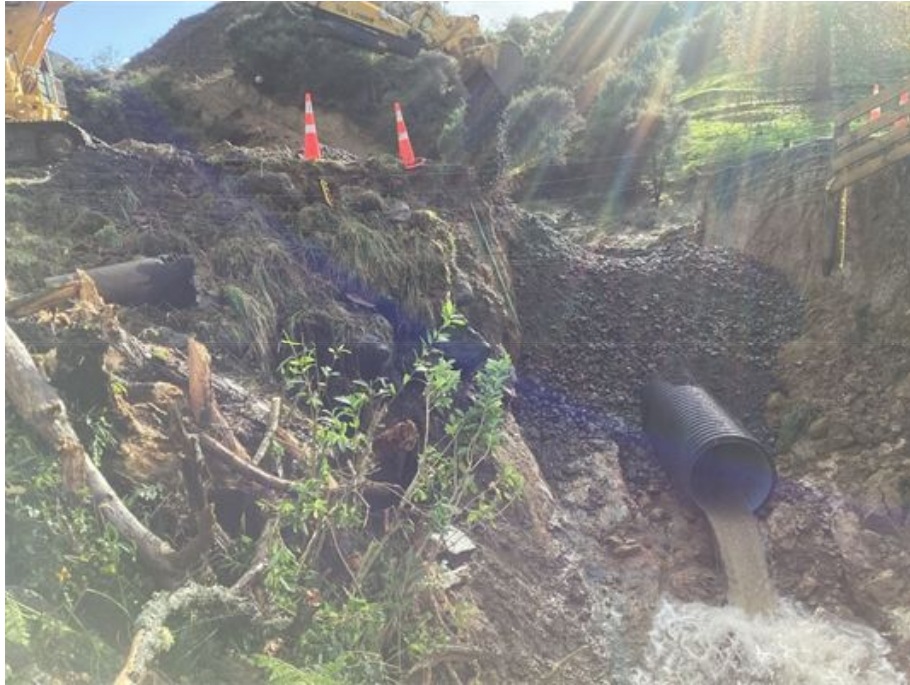
Figure 2: New culvert and backfill being installed to re-open the road
