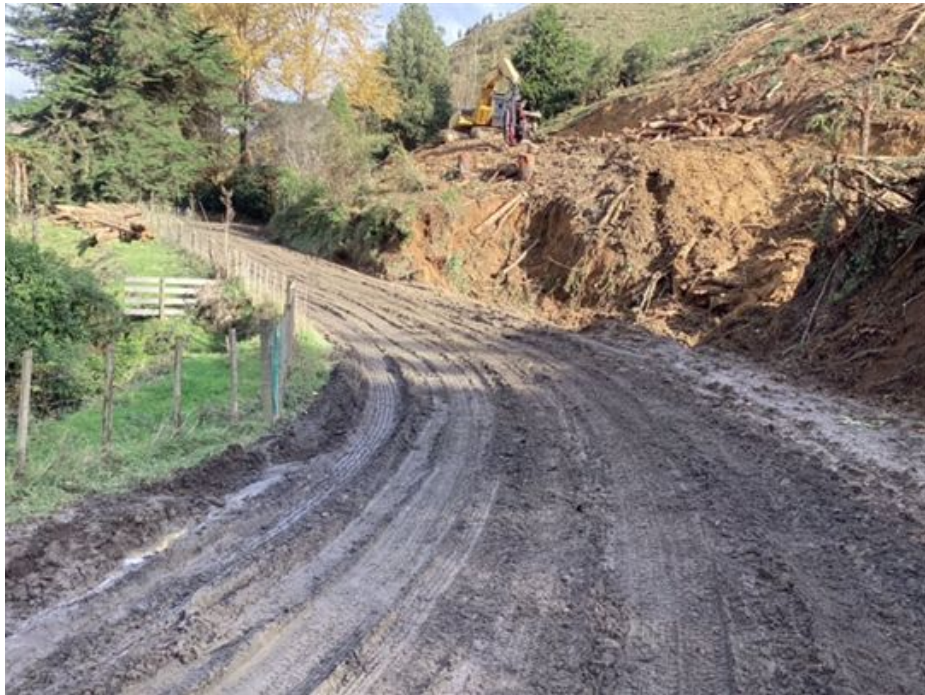
Figure 3: Condition of Upper Mangaehu Road as a result of logging in wet weather. Note the slash from the harvesting which is adjacent to a culvert
