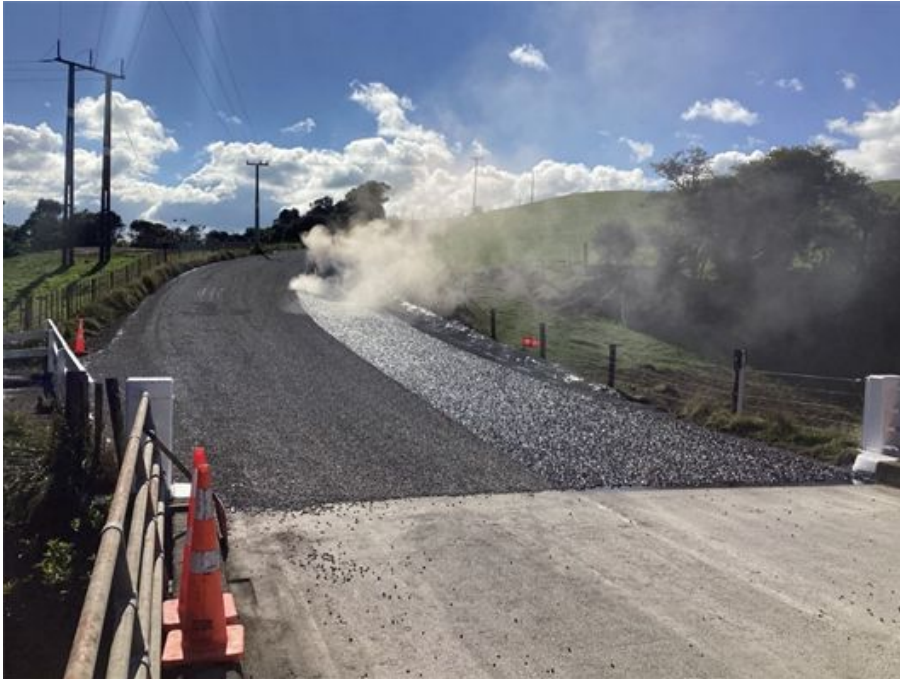
Figure 6: Palmer Road being sealed.
