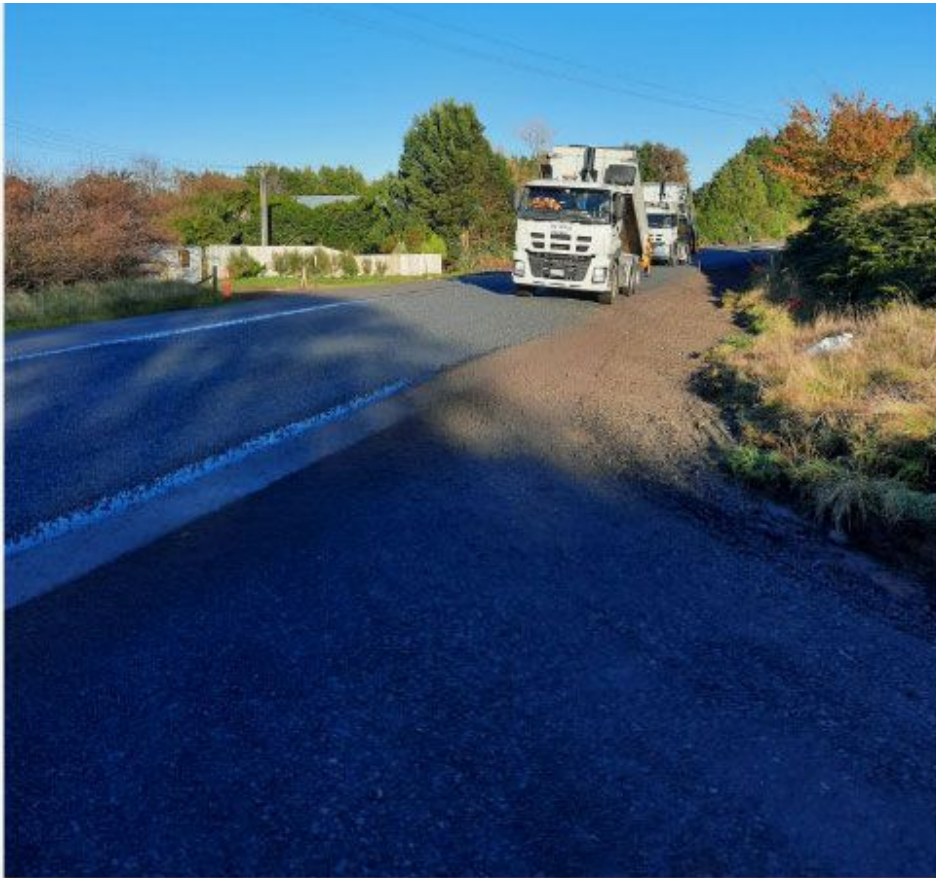
Figure 8: Sealing of Opunake Road
