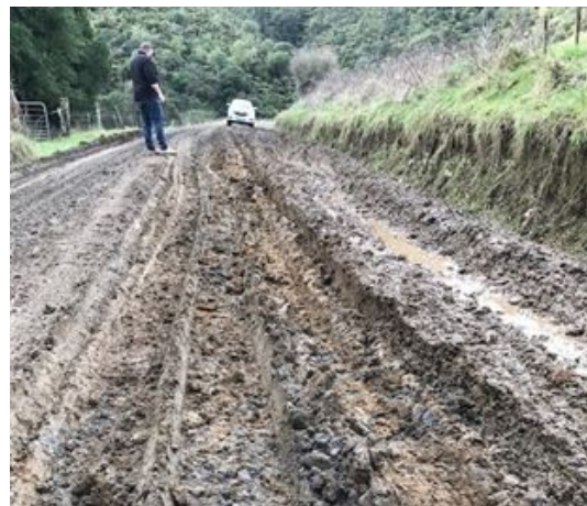
Above: A section of Puniwhakau Road is assessed.
