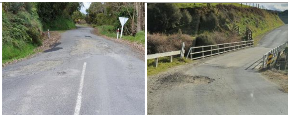
Figure 5: Examples of logging traffic damage at sealed intersections and bridge approaches. Left: Brewer Road/Upper Mangaehu Road intersection. Right: Mangaehu Road bridge approach seal
