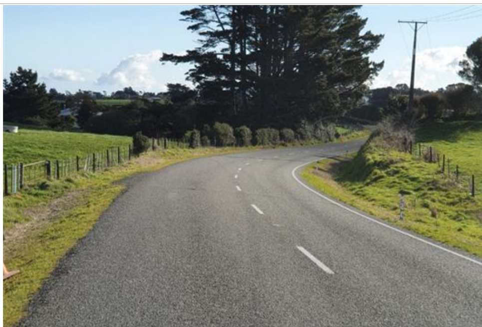
Figure 12: Non-compliant roadside delineation/application of edge marker posts, Opunake Road
