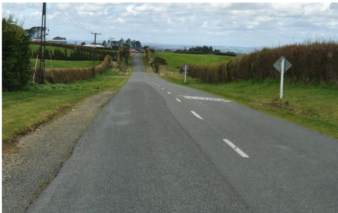
Figure 4: Monmouth Road, pavement rehabilitation and improvement project site
