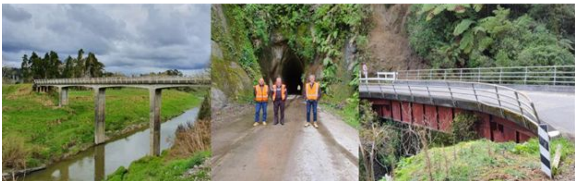
Examples of structures. Left: Junction Road bridge. Centre: Mangaoapa Road tunnel. Right: Matau Road bridge
