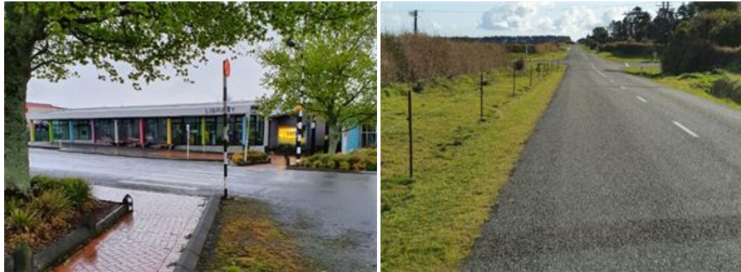
Figure 13: Examples of road safety deficiencies, pedestrian crossing with tactile pavers (left) and waratah standard temporary fencing (right).
