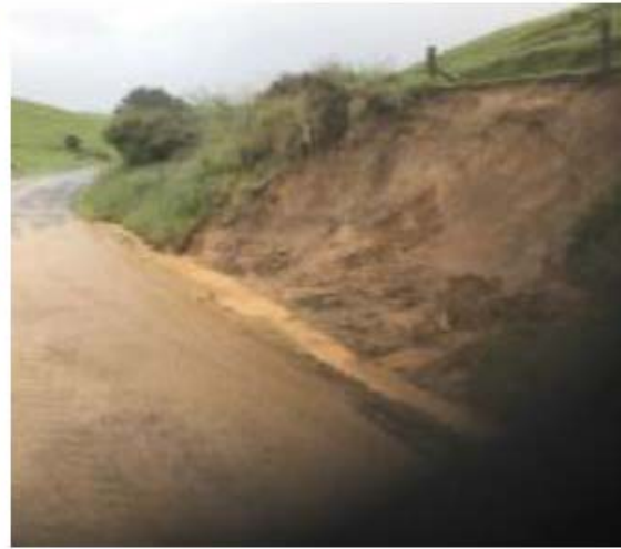
Wingrove Road - Slip Clearance
