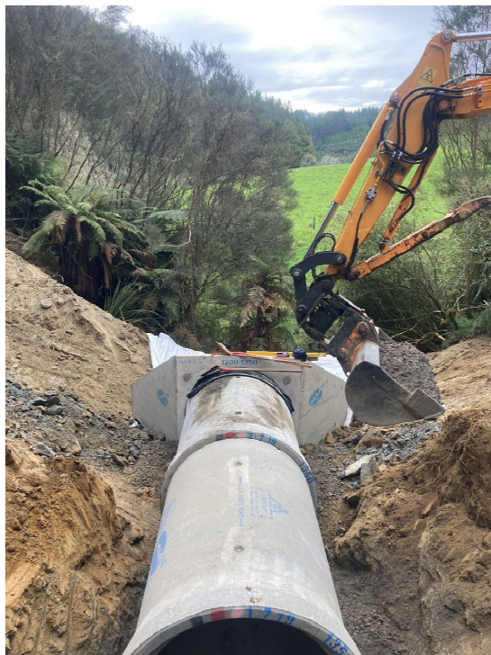
Figure 4: Culverts installed at the outlet
