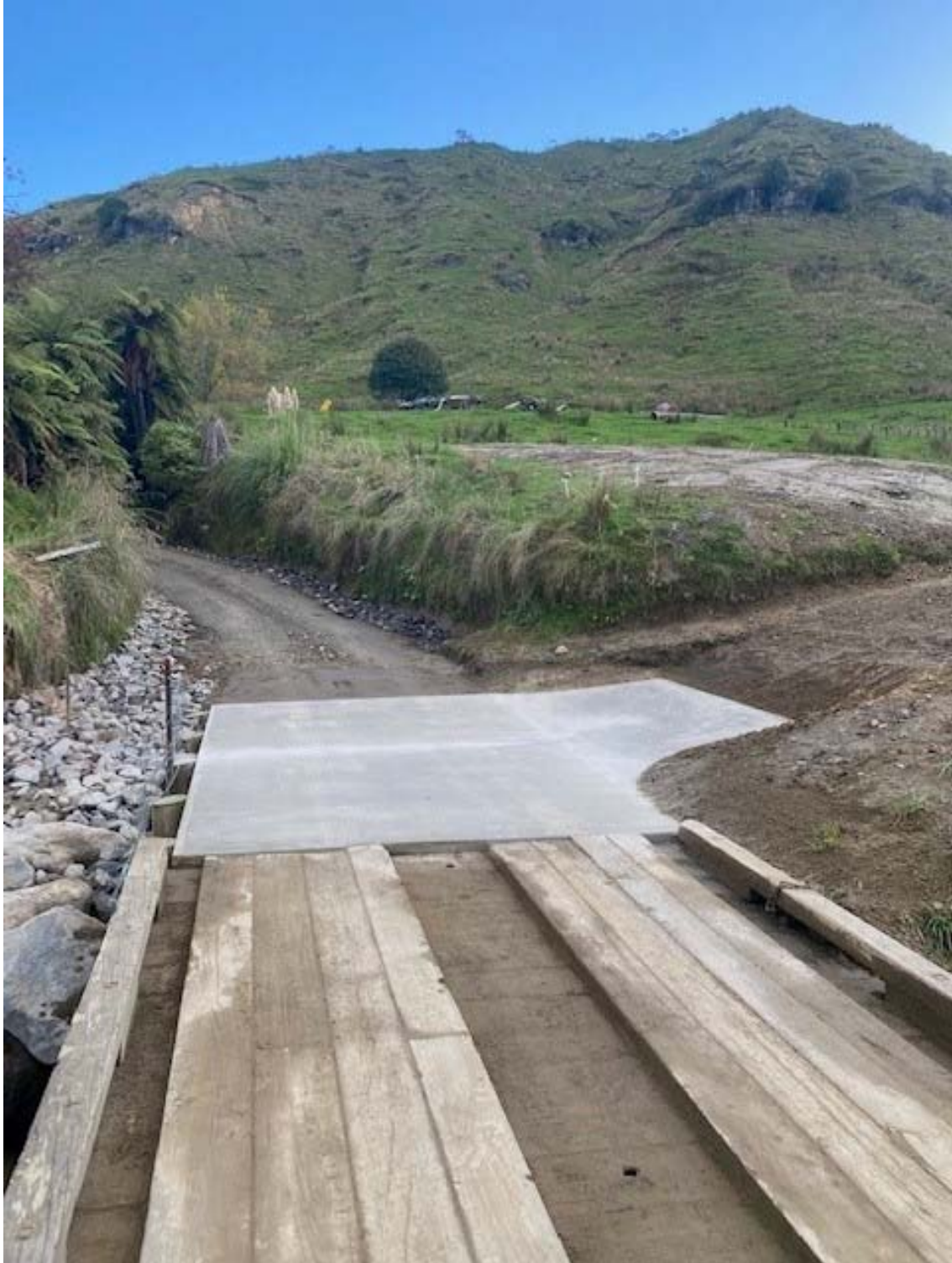
Figure 1- Repairs to the eastern approach to McBride's Bridge
