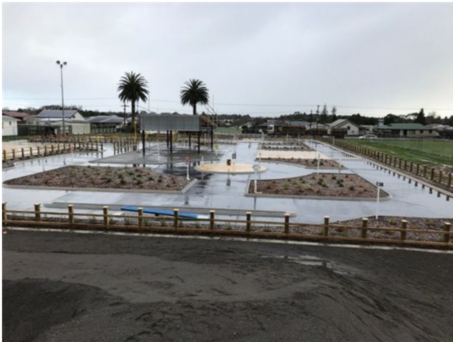
Figure 5: The Progress so far
