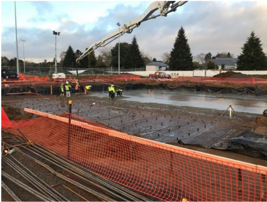
Figure 4: Slab construction at the pool site
